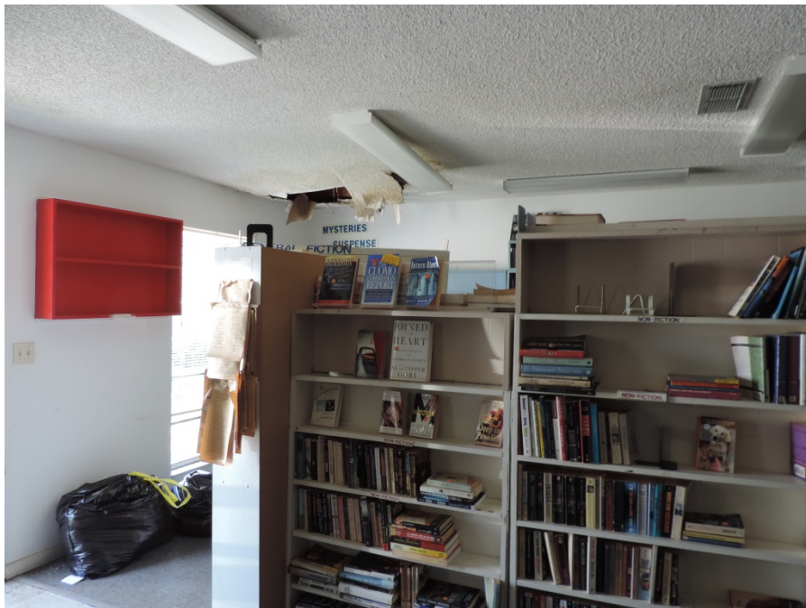
View of Retail Area
