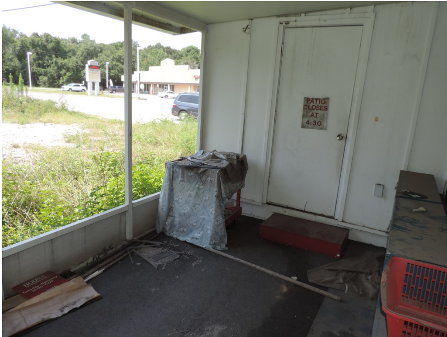
View of Screened Porch and Storage
