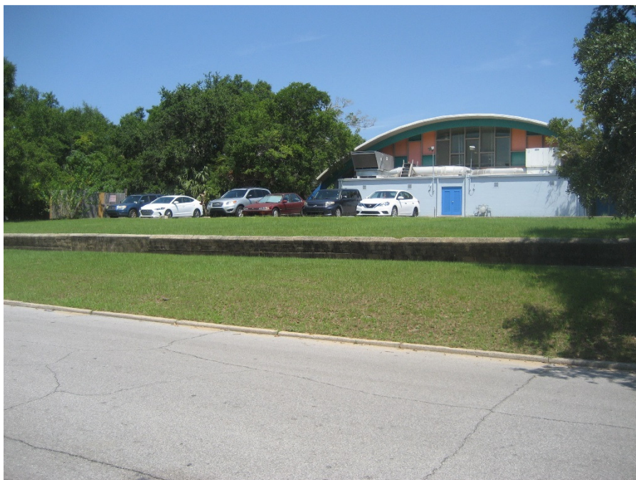
View of Rear of Subject Property From East La Rua Street
