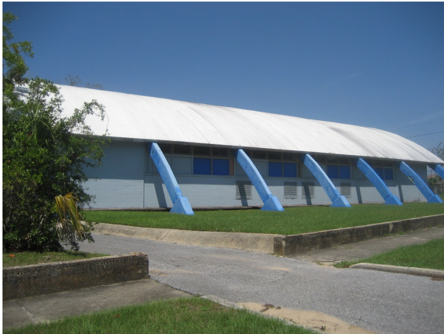
Side View of Subject Building
