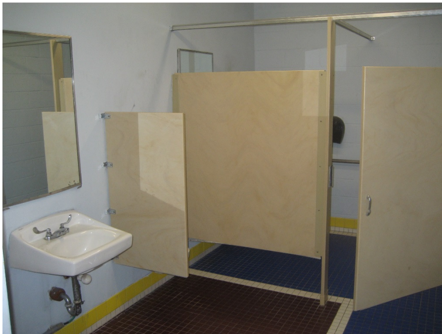
View of Typical Restroom in Subject Building
