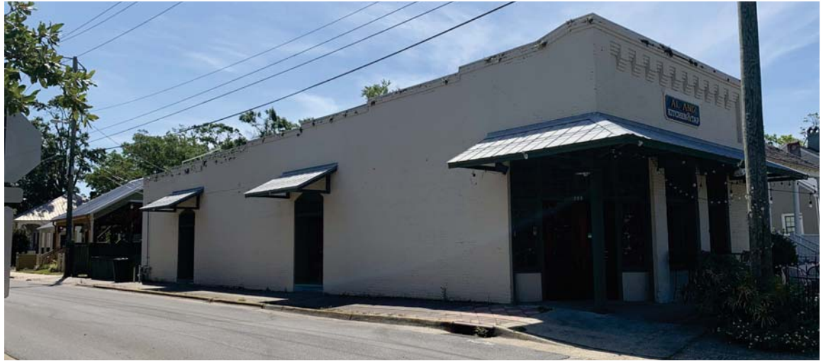
EAST INTENDENCIA STREET EXISTING PHOTO
