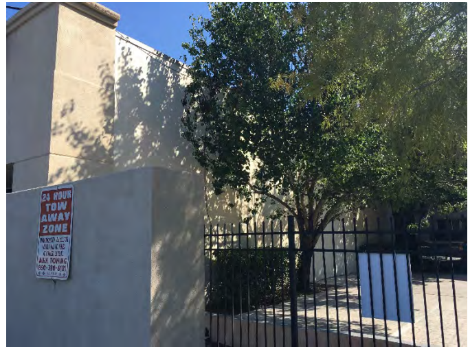
View of Existing South Side
