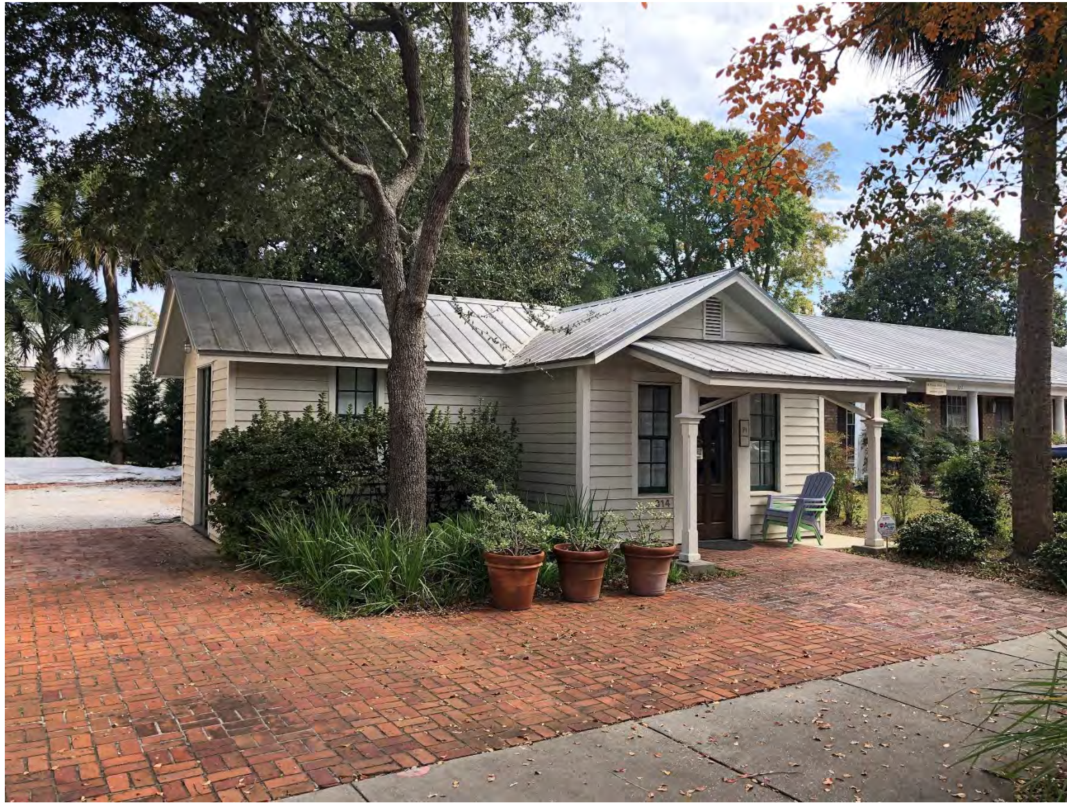
FRONT VIEW LOOKING SE
