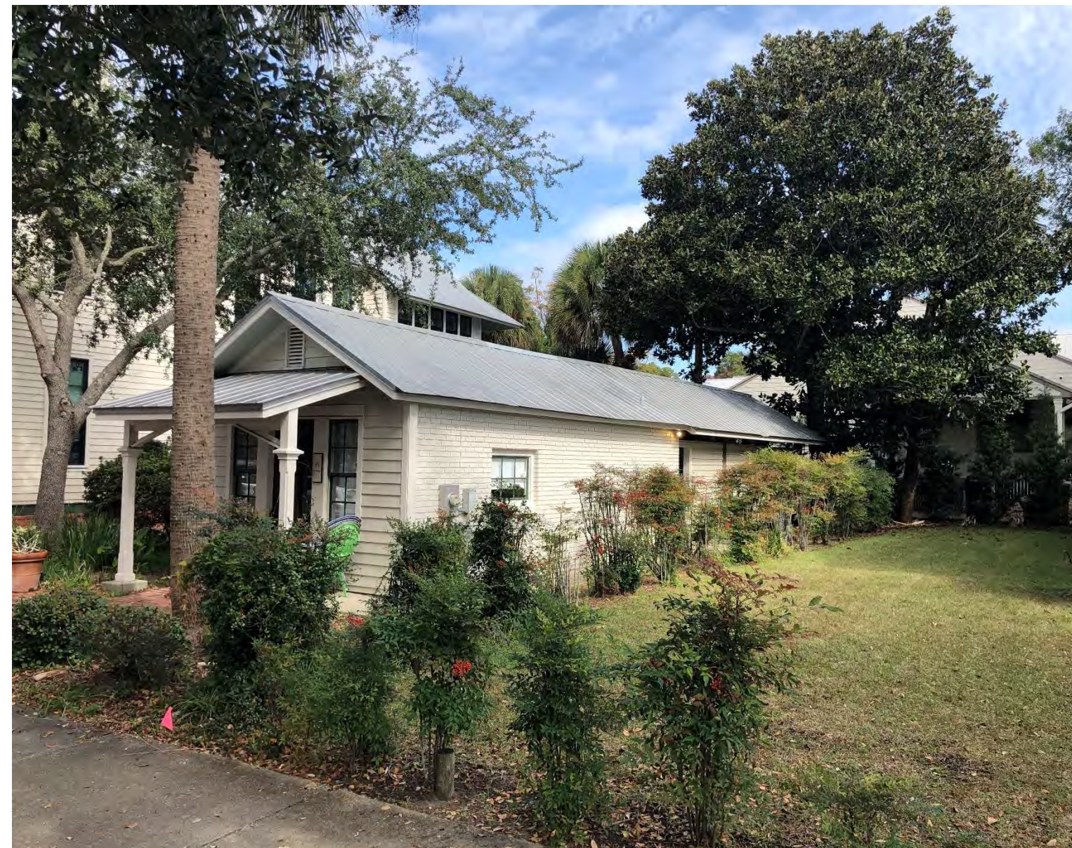
FRONT VIEW LOOKING NE
