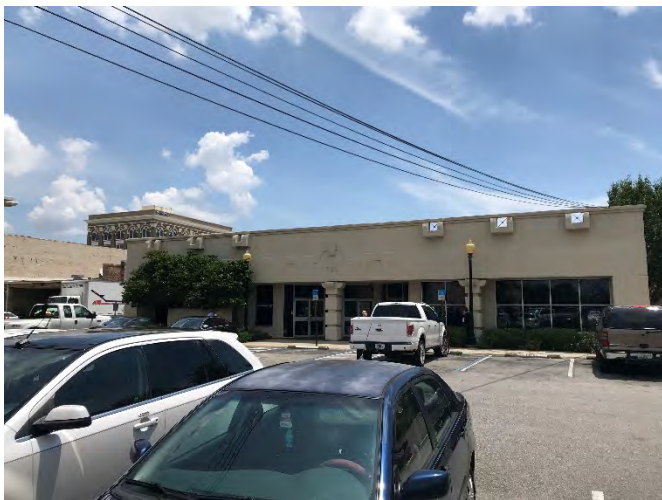
View of Existing Rear
