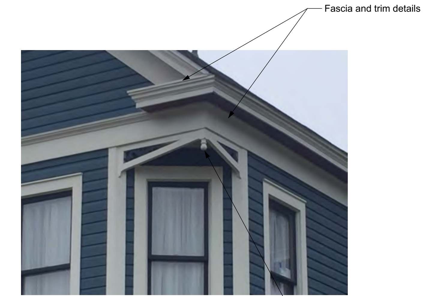
Fascia and trim details
