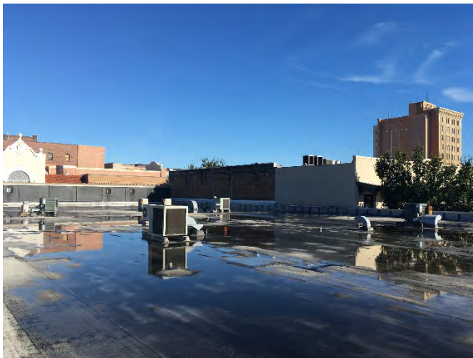
View of Existing Roof
