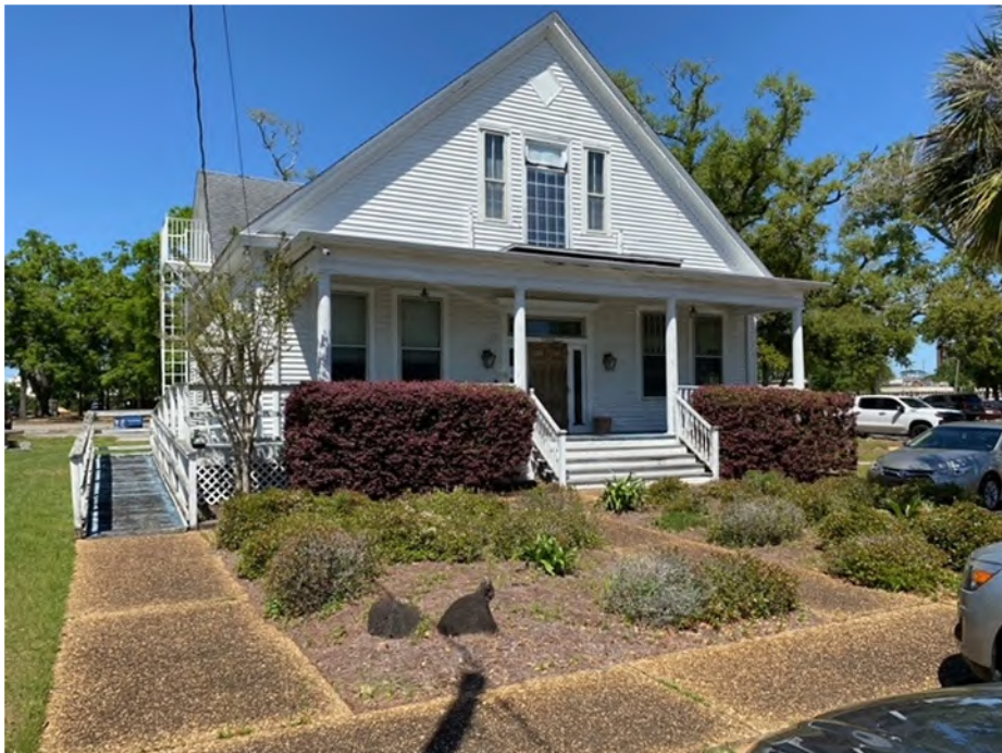
Front View of Subject Building – Office Property (Parcel A)
