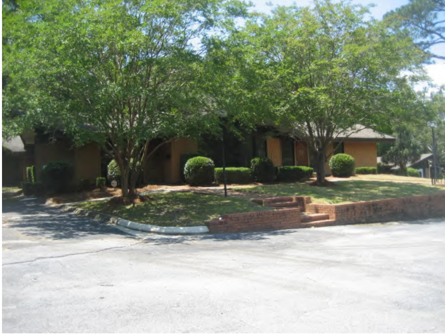
(8817) 4709 Scenic Highway, Pensacola, Florida
