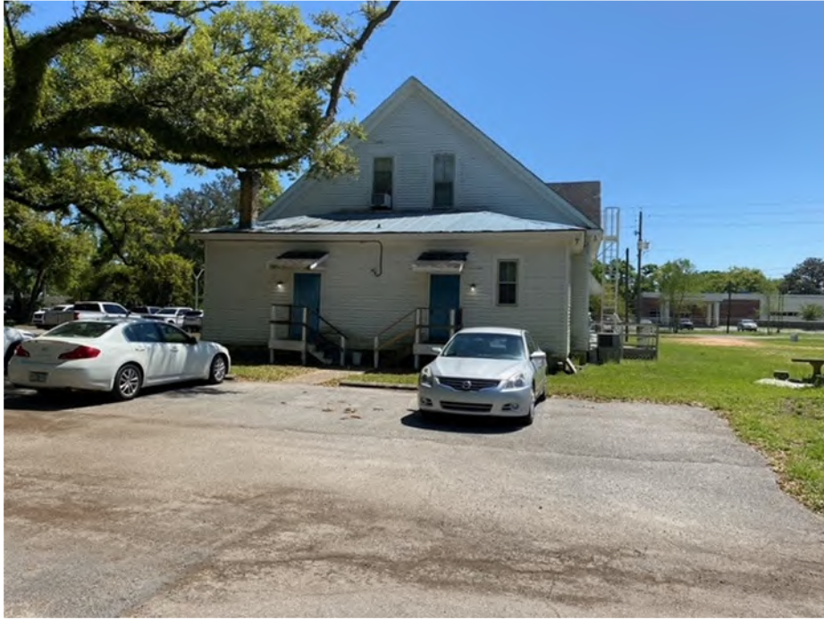
Rear View of Subject Building – Office Property (Parcel A)
