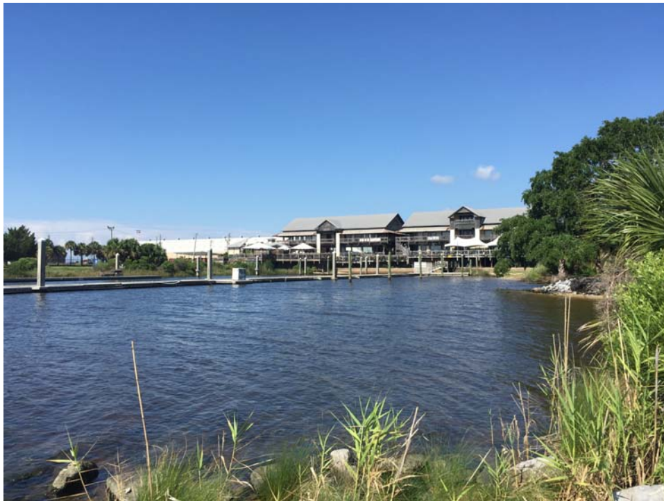
View of Subject Property Eastern Building Side and Damaged Marina
