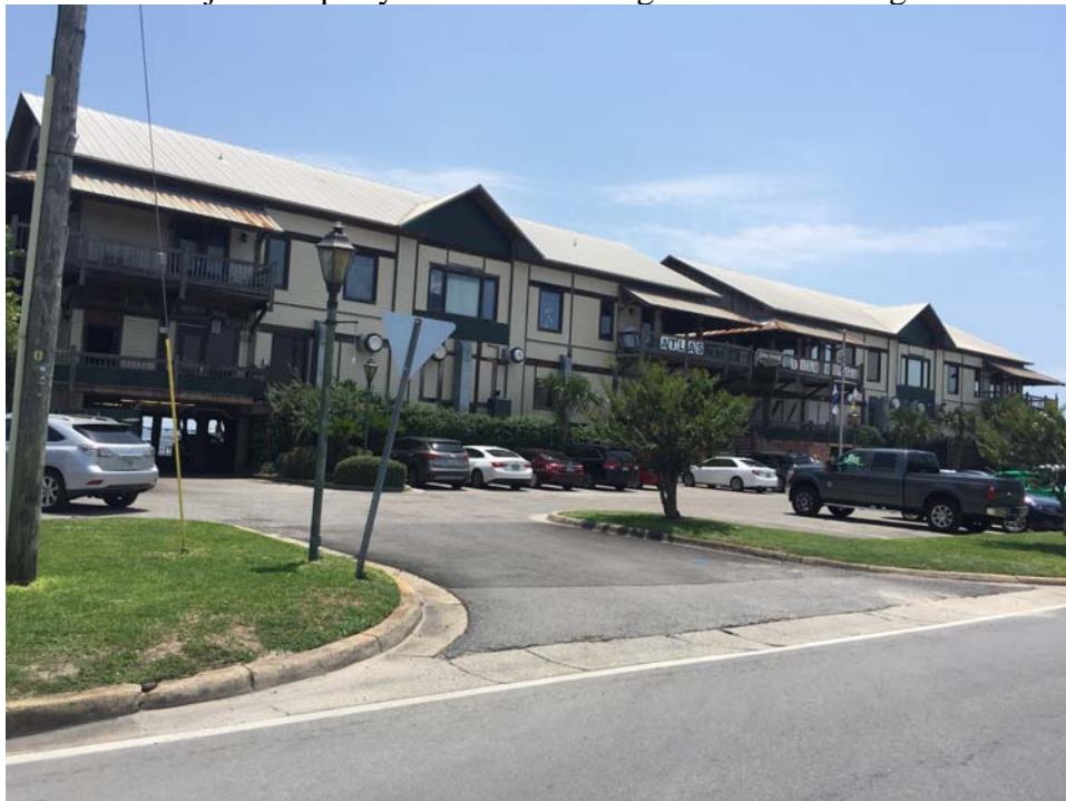
View of Subject Property Western Building Side
