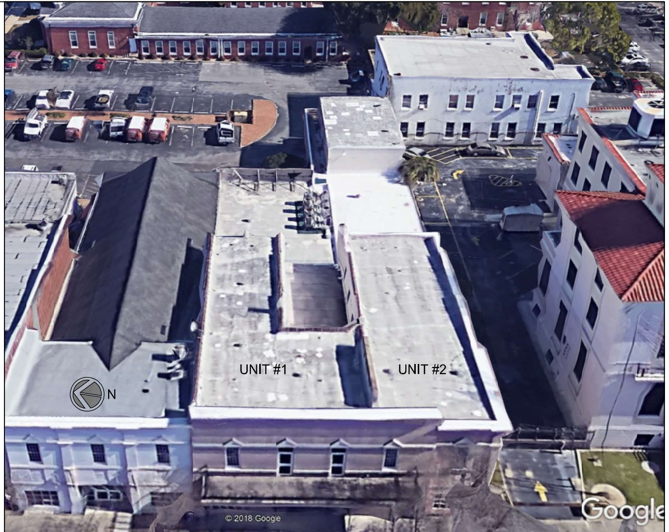
AERIAL VIEW / FRONT OF BUILDING
