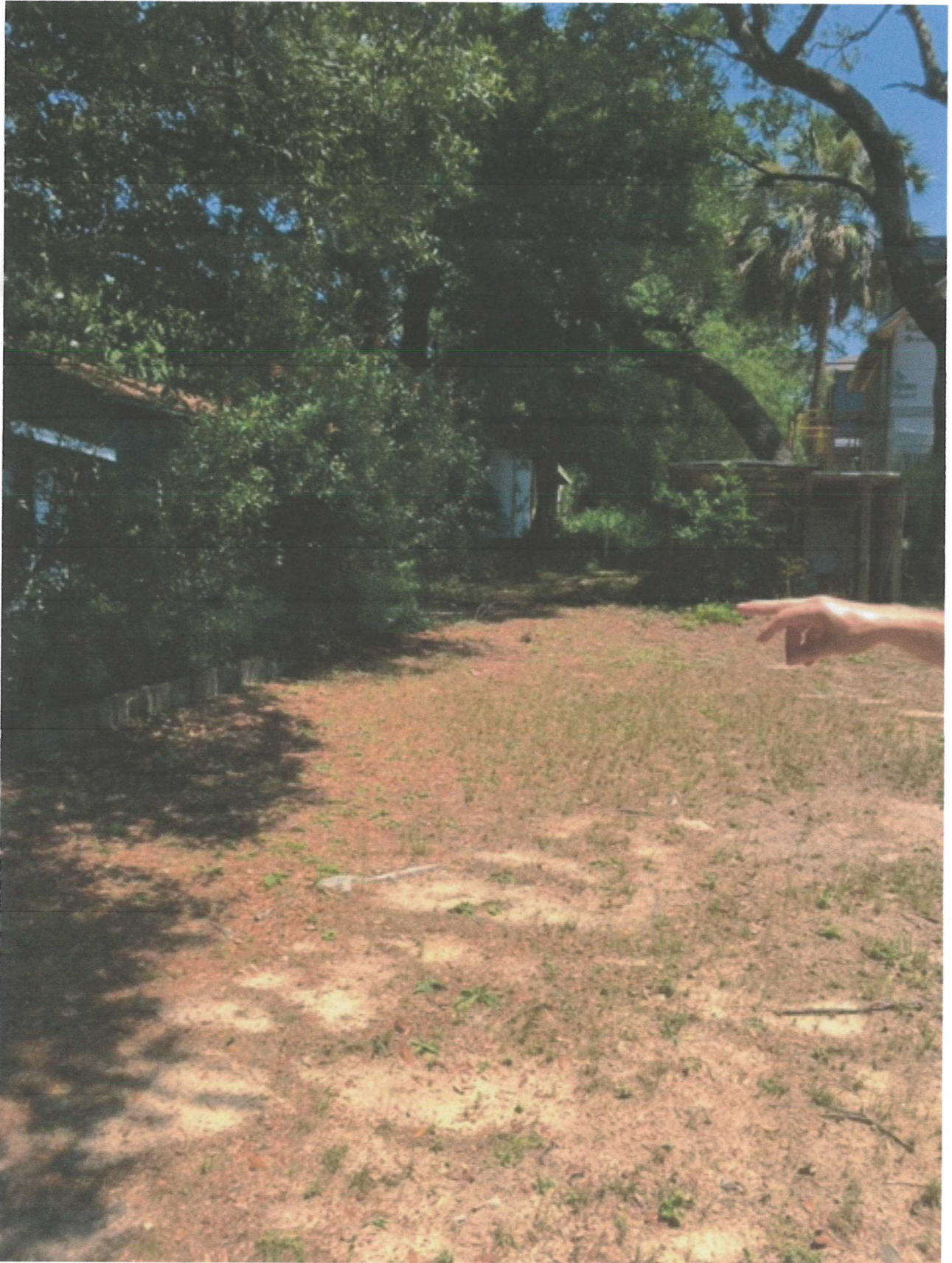
CINDERBLOCK RETAINING WALL BUILT THROUGH ALLEY
