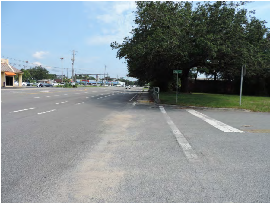
View North on Tippin Avenue
