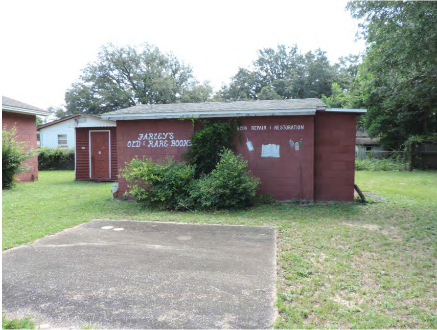
View of Concrete Block Storage Building
