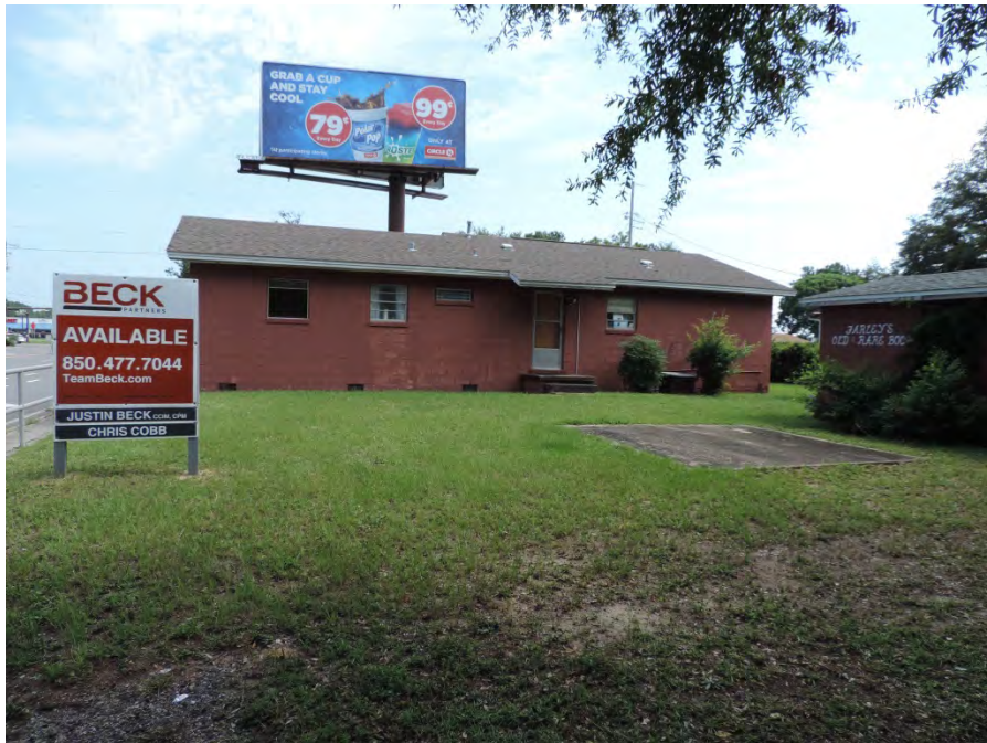
Rear Exterior View of Improvements
