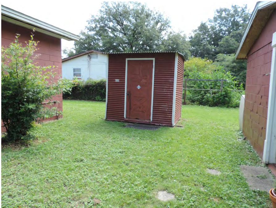
View of Small Metal Storage Building
