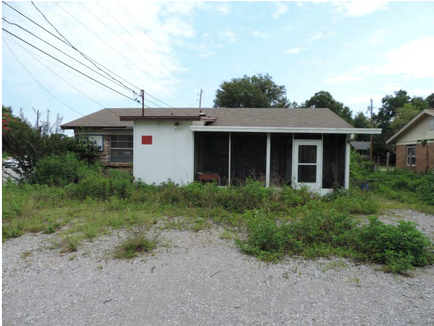
Rear Exterior View of Improvements
