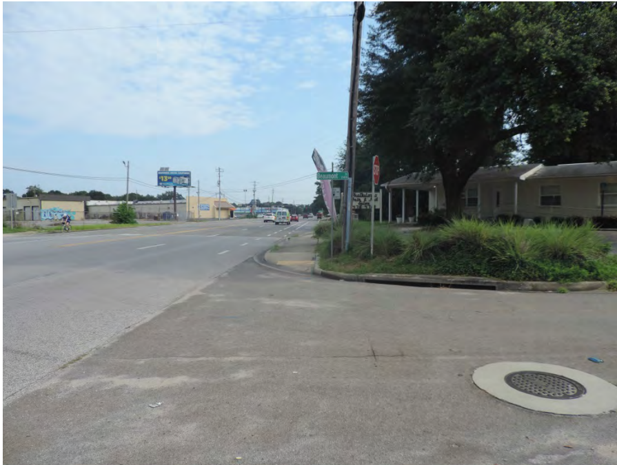
View North on Tippin Avenue
