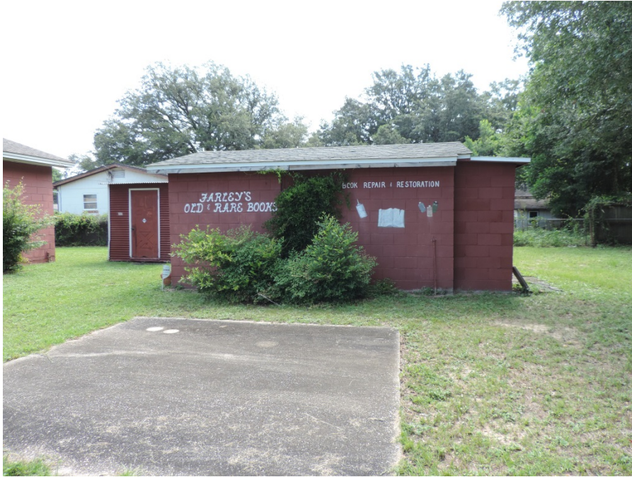
View of Concrete Block Storage Building
