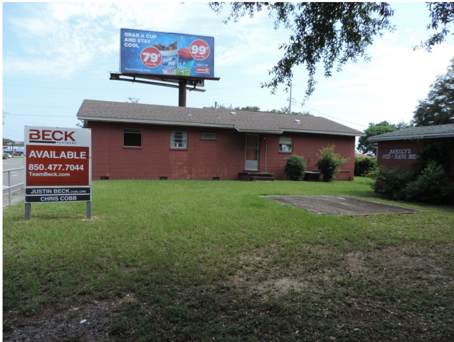
Rear Exterior View of Improvements
