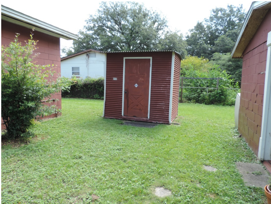
View of Small Metal Storage Building
