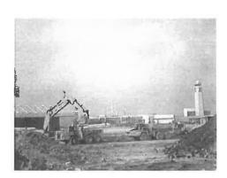
exceeded 24 tons. Three storm structures were too large to precast, so IX concrete crews were enlisted to cast them in place. In addition to the pipe work, the storm system included excavation of an 118,000 CY dry pond with a paved concrete gutter, 271 LF of 48" bored and jacked underneath Brookpark Road and the re-building of the North Detention Basin located north of I-480 off Grayton Road.
