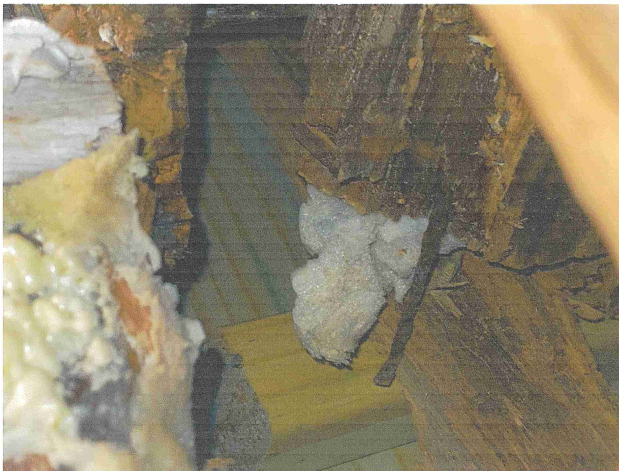
Close up of rotted stud "holding" up the door.
