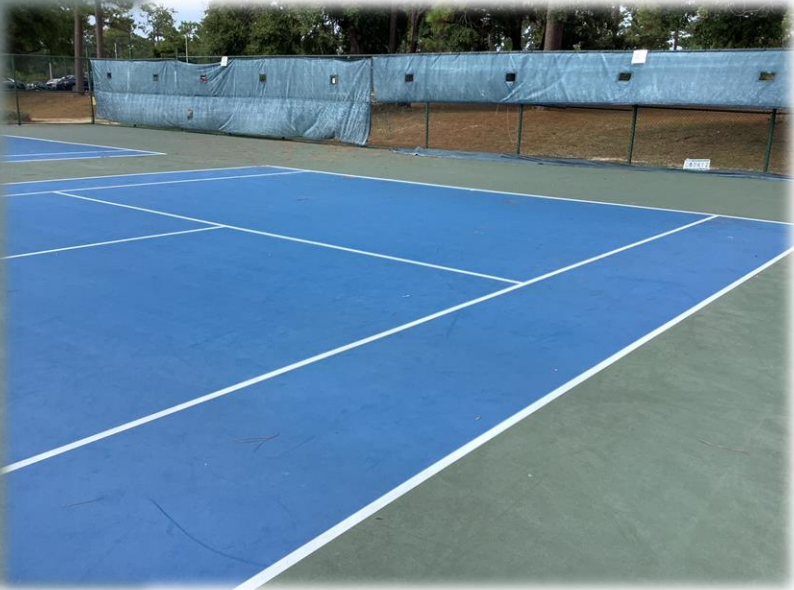
UWF post tension court #2 October 2022
