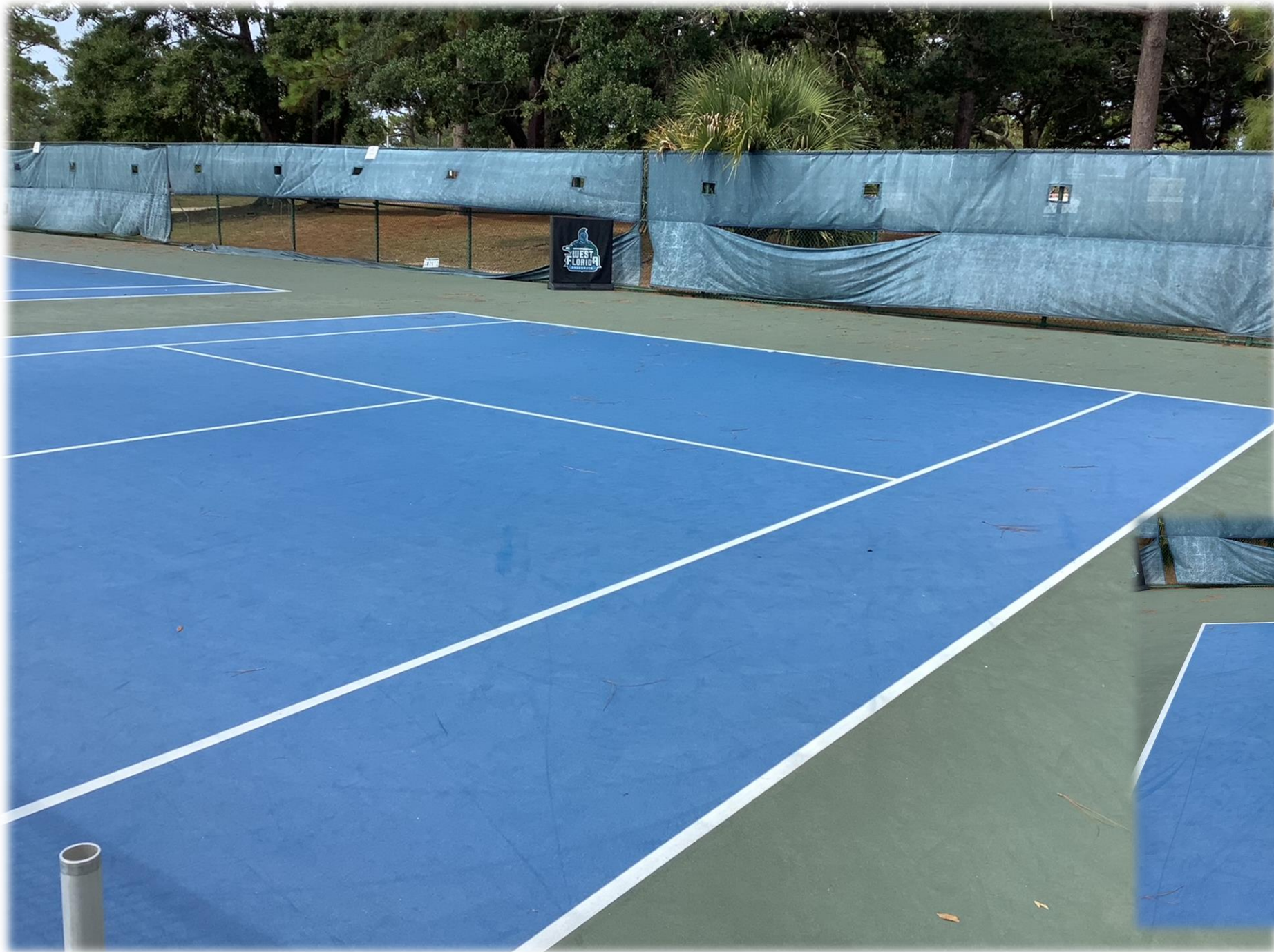
UWF post tension court #3 October 2022
