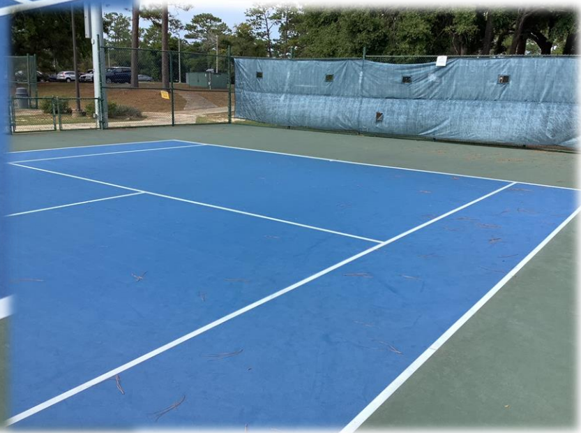
UWF post tension court #3 October 2022
