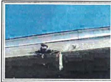
Subject: Roof eave damage on rear
