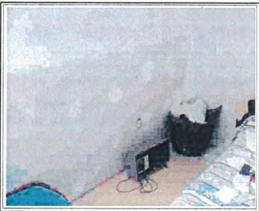
Subject: Right Side Bedroom- Missing outlet cover and unfinished painting
