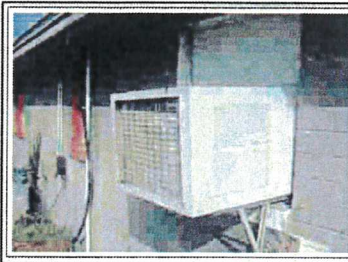
Subject: Through wall H/A unit in left front bedroom
