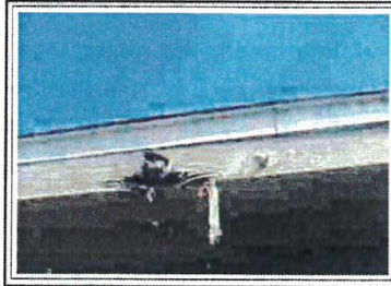
Subject: Roof eave damage on rear
