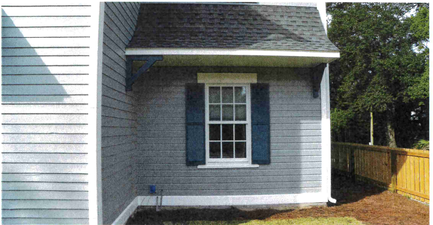
Photo 2 – Restored base of tower that was previously an entry and small room. 10/28/16
