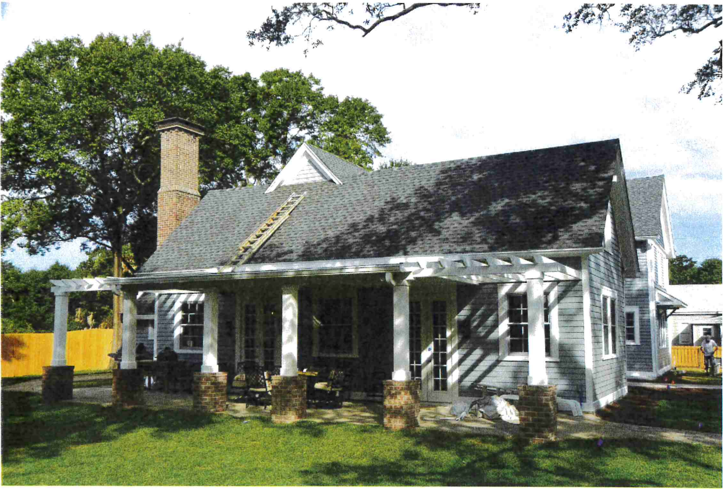
Photo 7 – Restored south façade (rear of the house). 10/28/16
