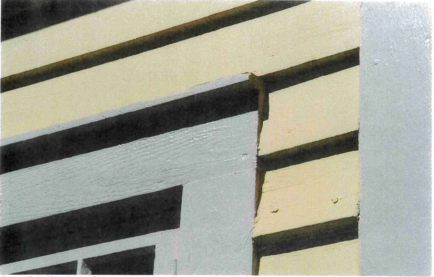
Photo 7-1 - Wood Lap Siding and Trim
