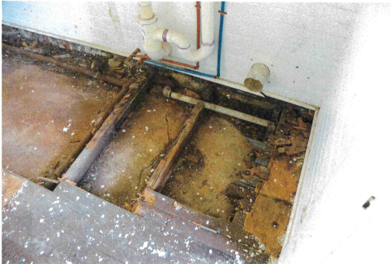
Photo 2 - 1st Floor Flooring
