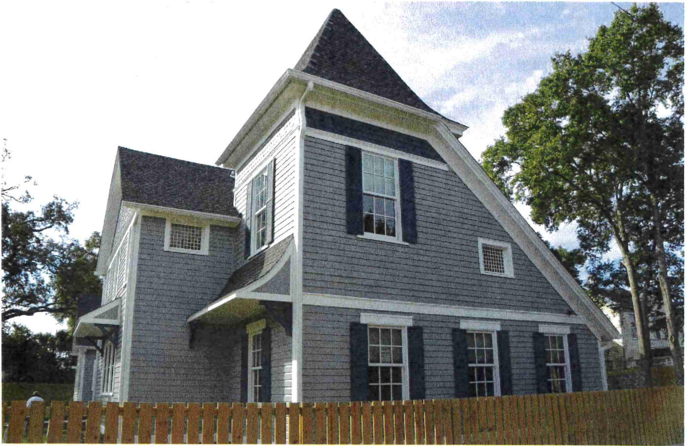
Photo 3 – Restored north façade. 10/28/16
