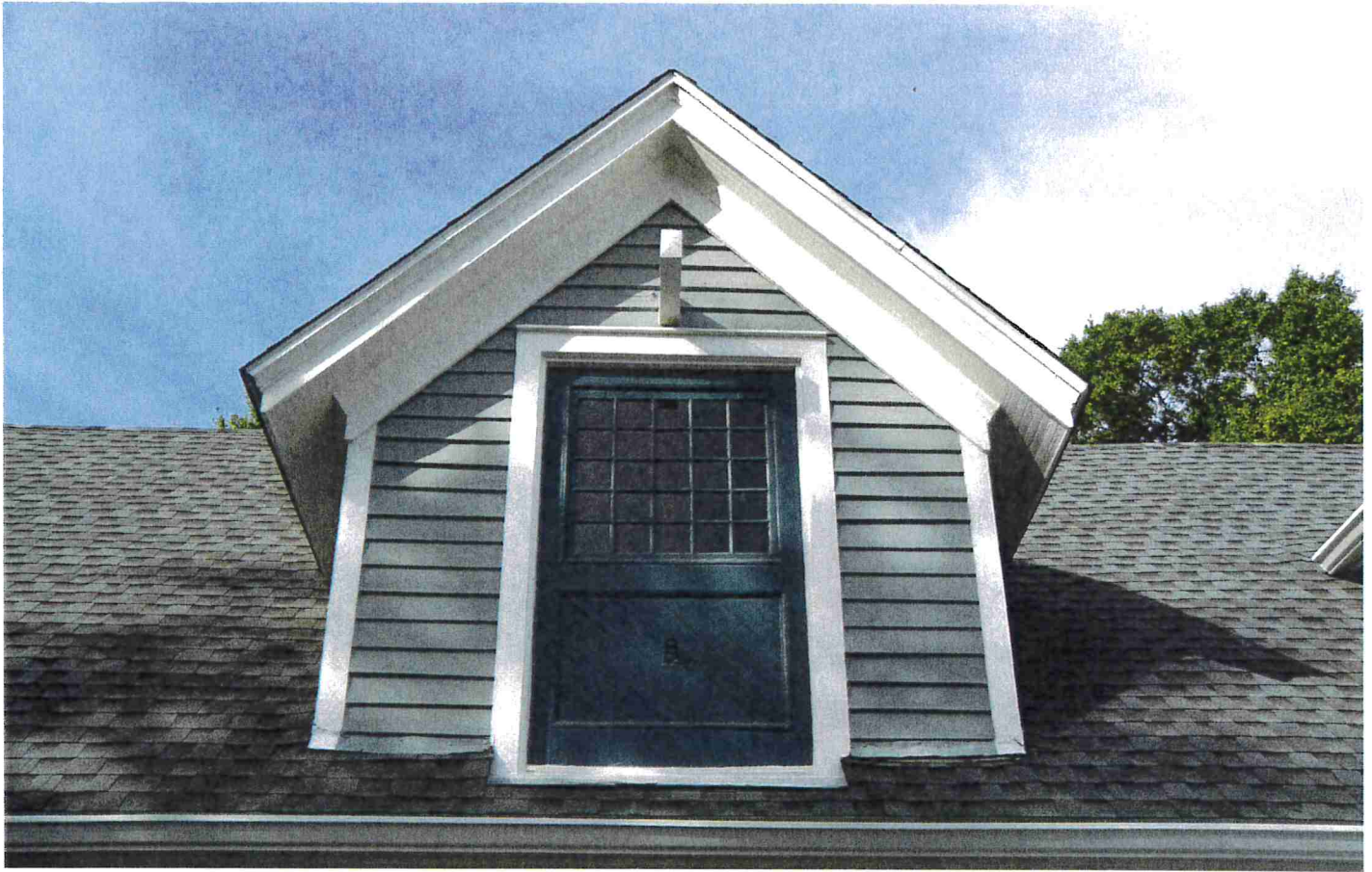
Photo 15 – Restored dormer above entry on east façade. 10/28/16
