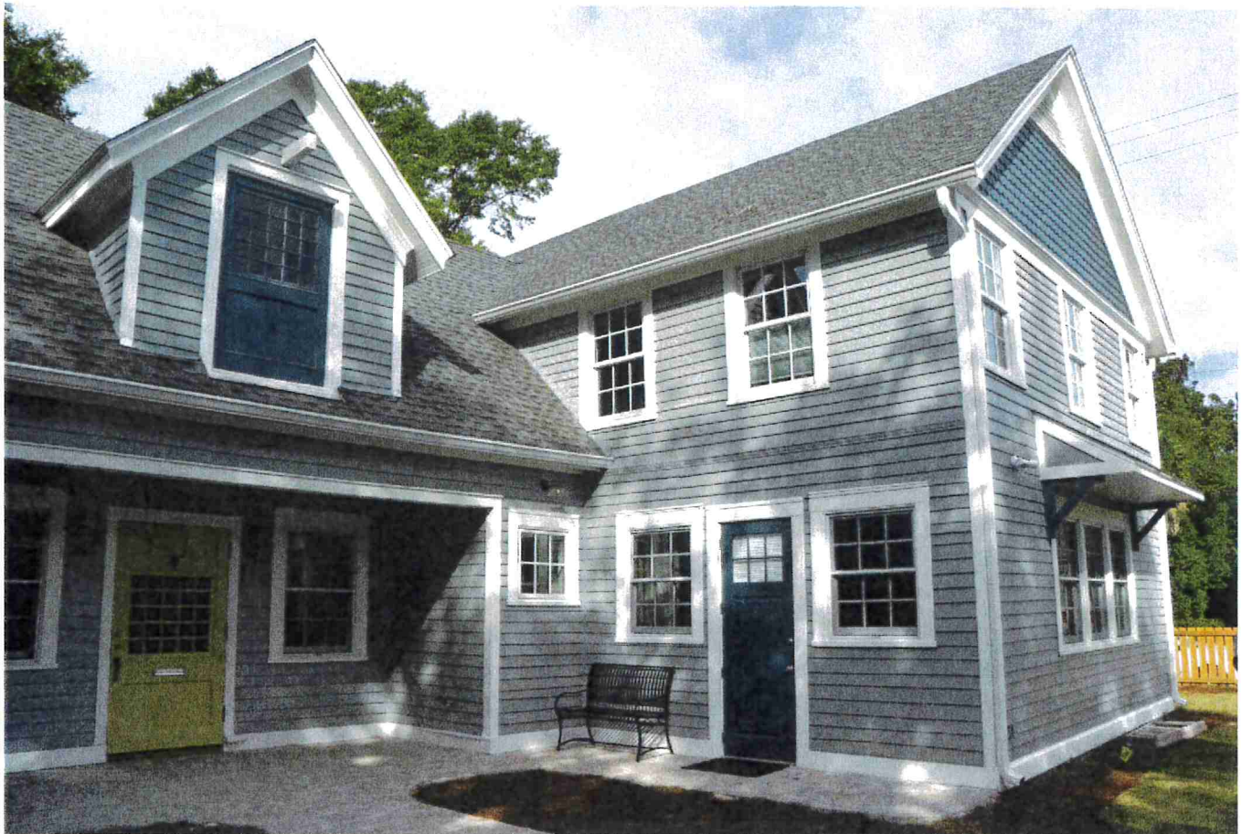
Photo 10 – Restored east façade and main entrance. 10/28/16
