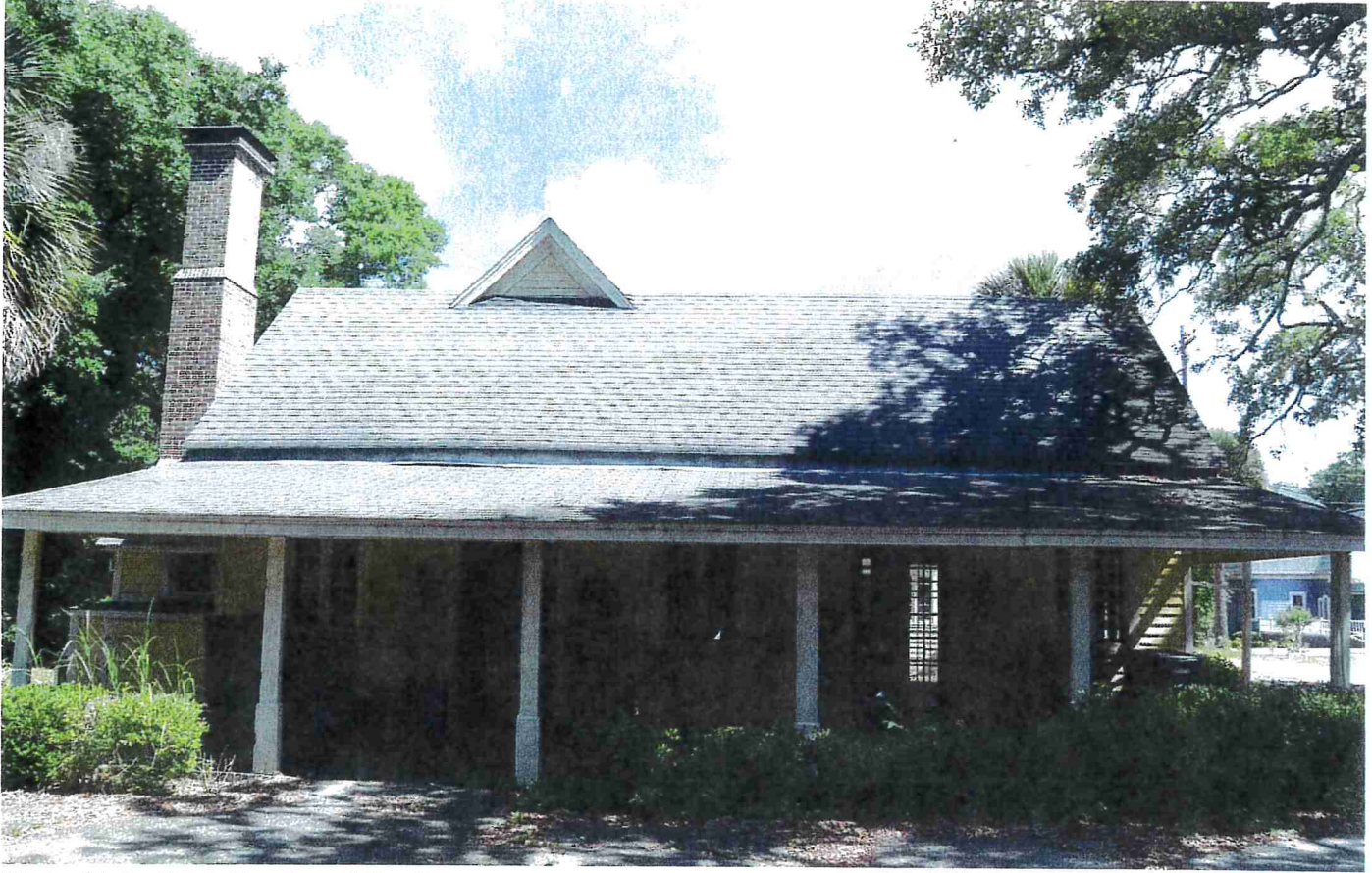
Photo 11-1 - Brick Porch and Roof
