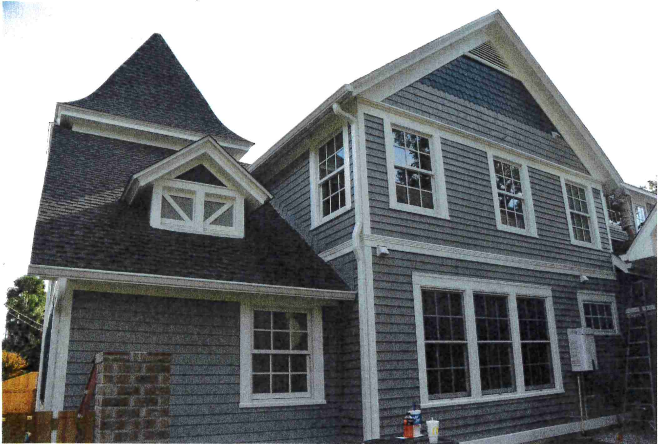
Photo 4 – Restored west façade with pervious sunroom addition removed. 10/28/16
