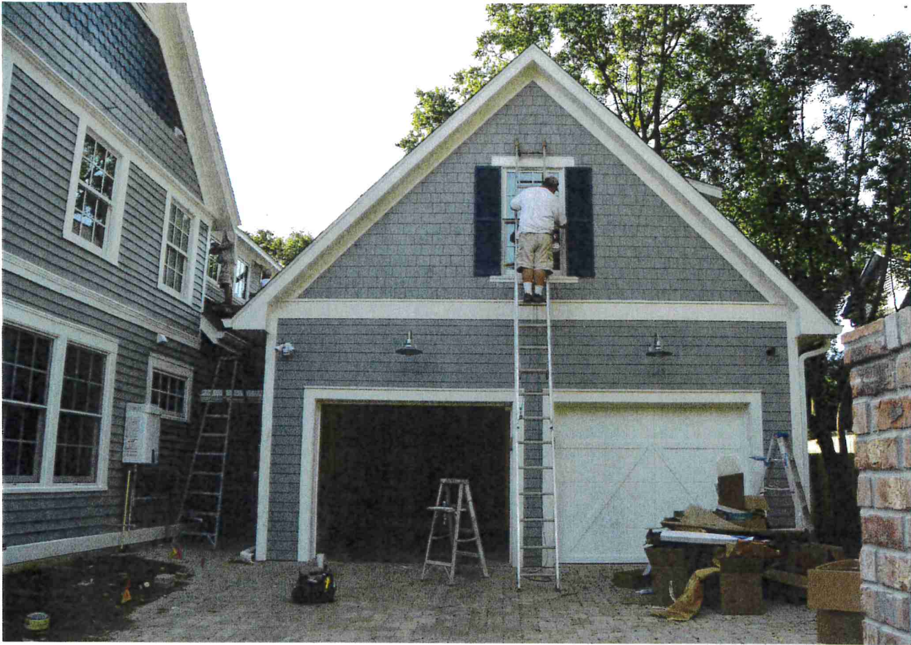
Photo 5 – New garage addition. 10/28/16
