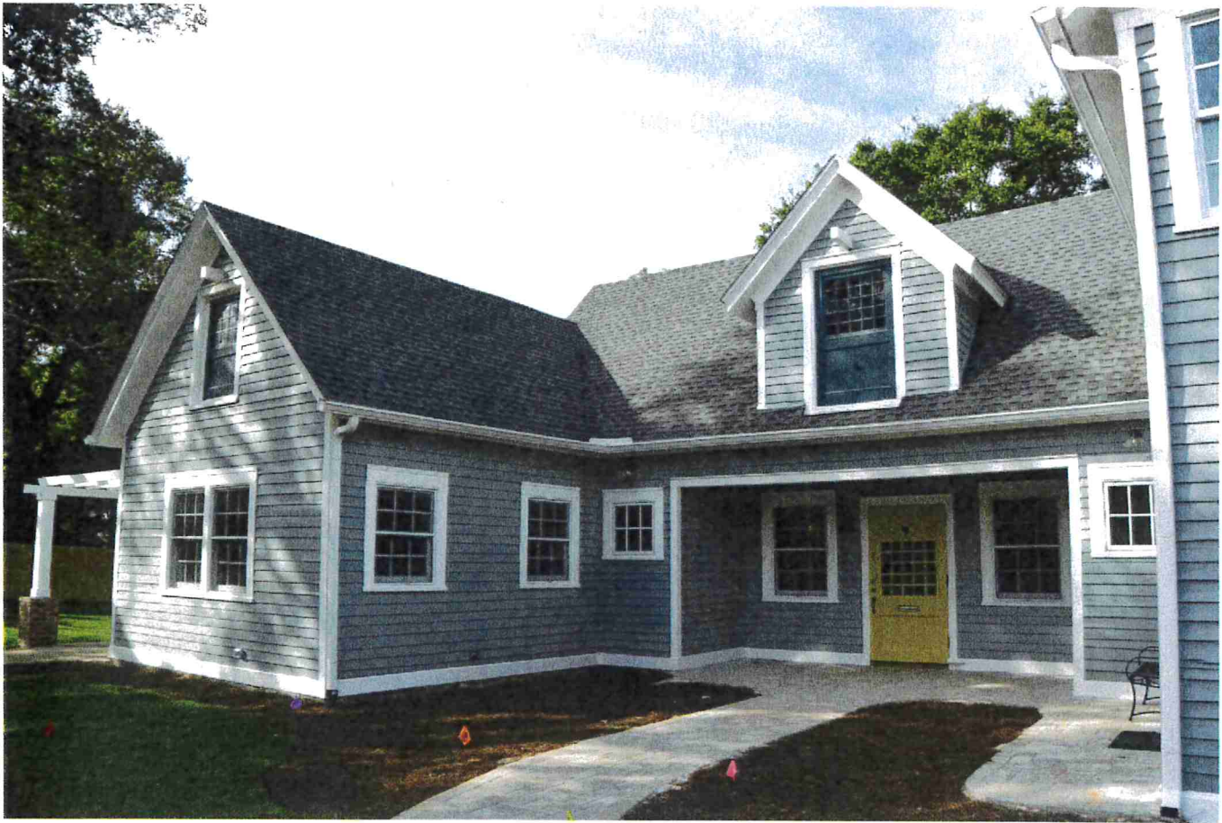
Photo 9 – Restored east façade and main entrance. 10/28/16
