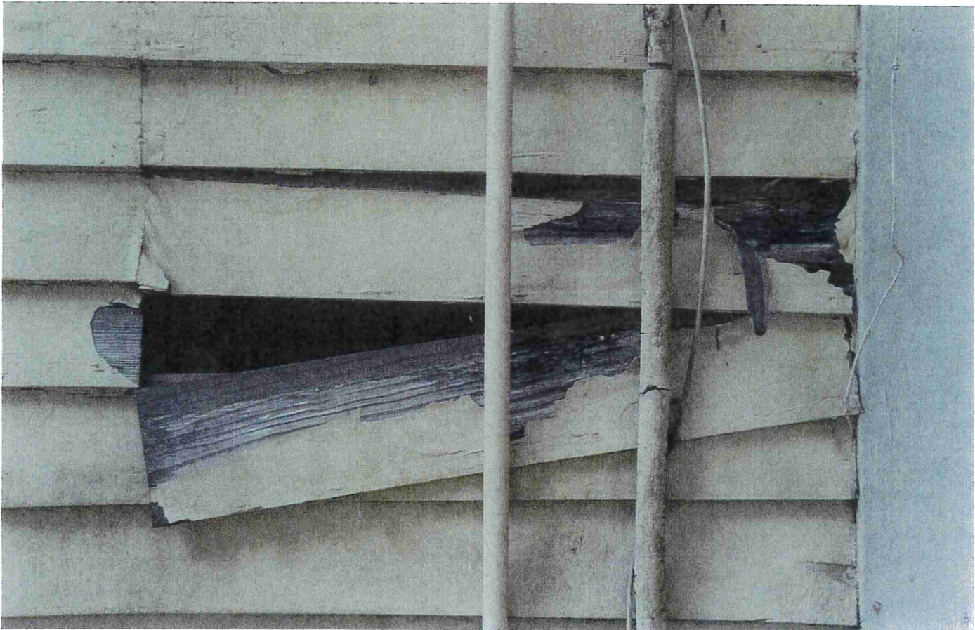
Photo 7-2 - Wood Lap Siding and Trim
