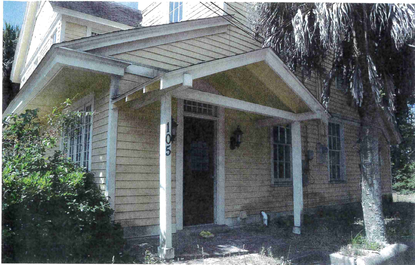
Photo 3 - Low Slope Entry Roof and Entry
