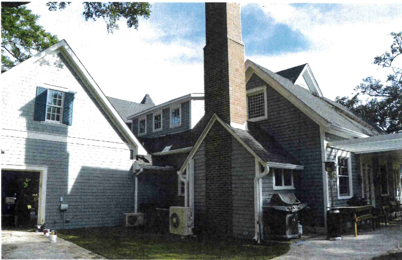
Photo 6 – Restored west façade (rear of the house). 10/28/16
