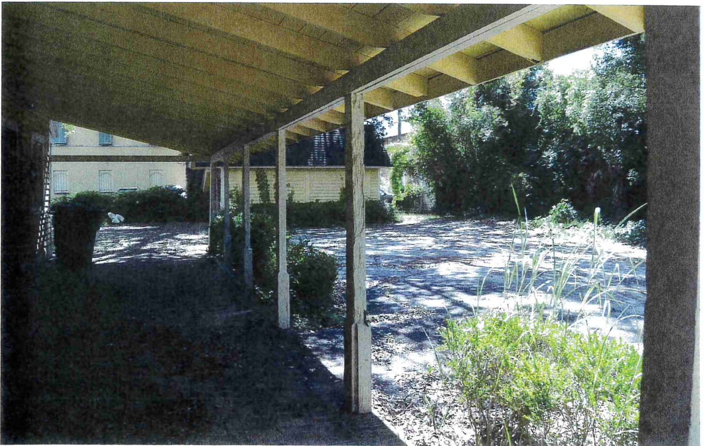
Photo 11-2 - Brick Porch and Roof
