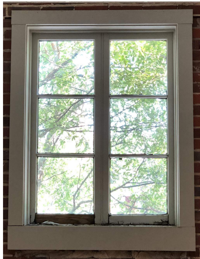
EXISTING UPPER WINDOW TO BE REPLACED (INTERIOR VIEW)
