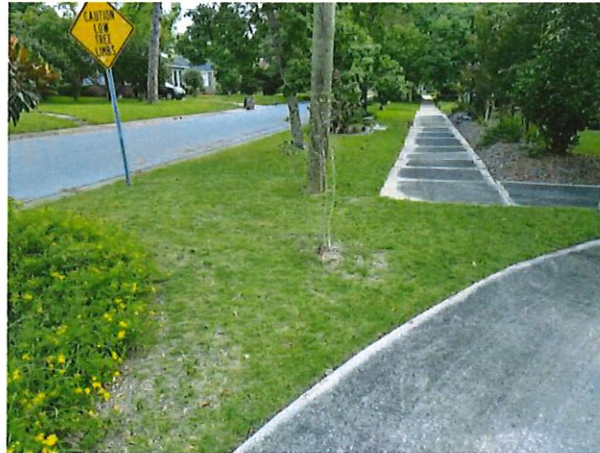
(Above) The sidewalk on the right of way at 18 th and Moreno does not connect to the street or the other side of the street.
