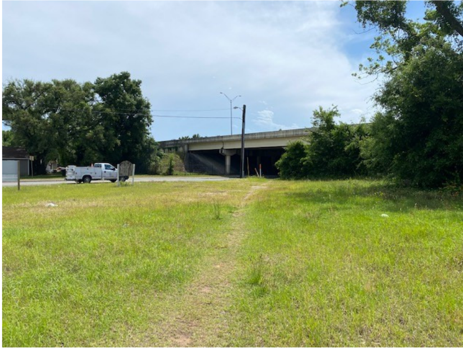
View of Interior of Subject Parcel
