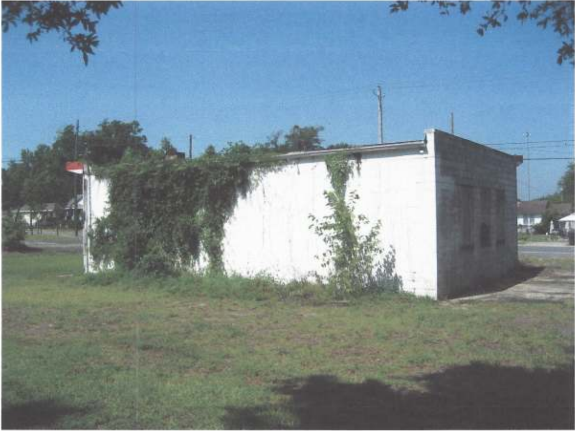
View of Rear of Subject Building
