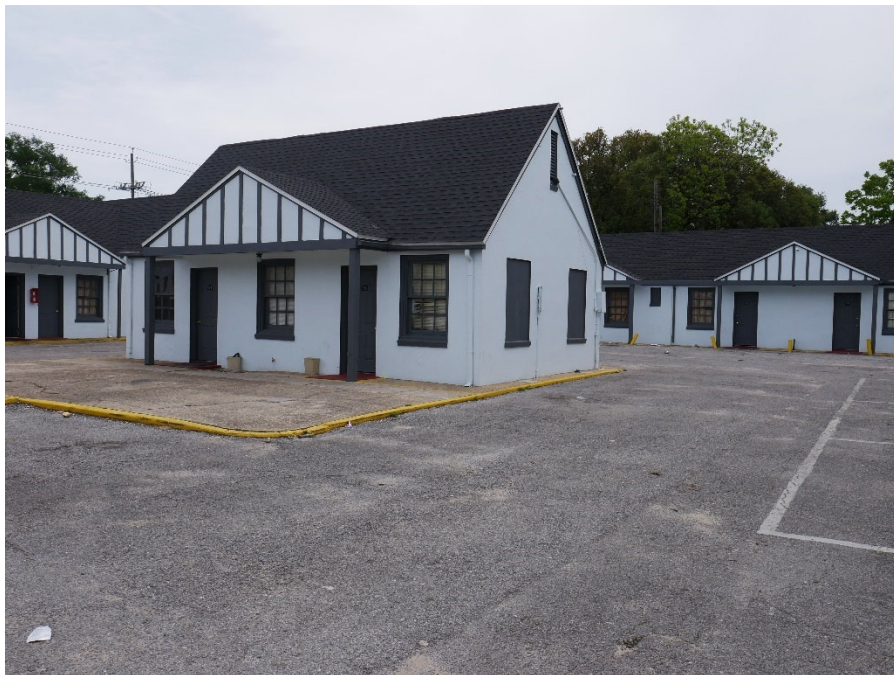
Front Exterior of Units 122 and 123
