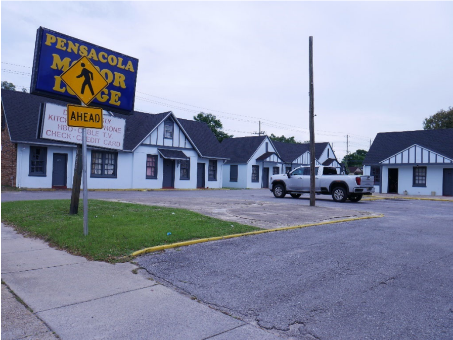
Front Exterior View of Improvements
