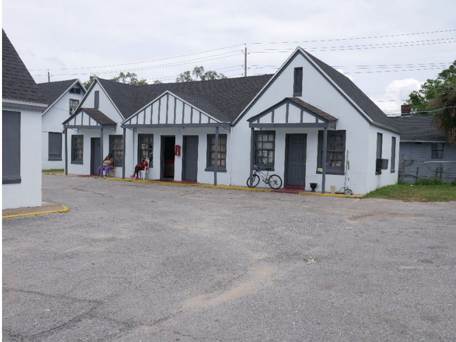
Front Exterior of Units 105, 106, 107 and 108
