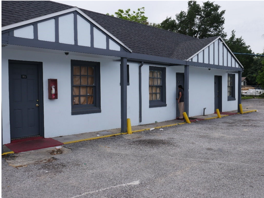
Front Exterior of Building with Units 114 thru 117
