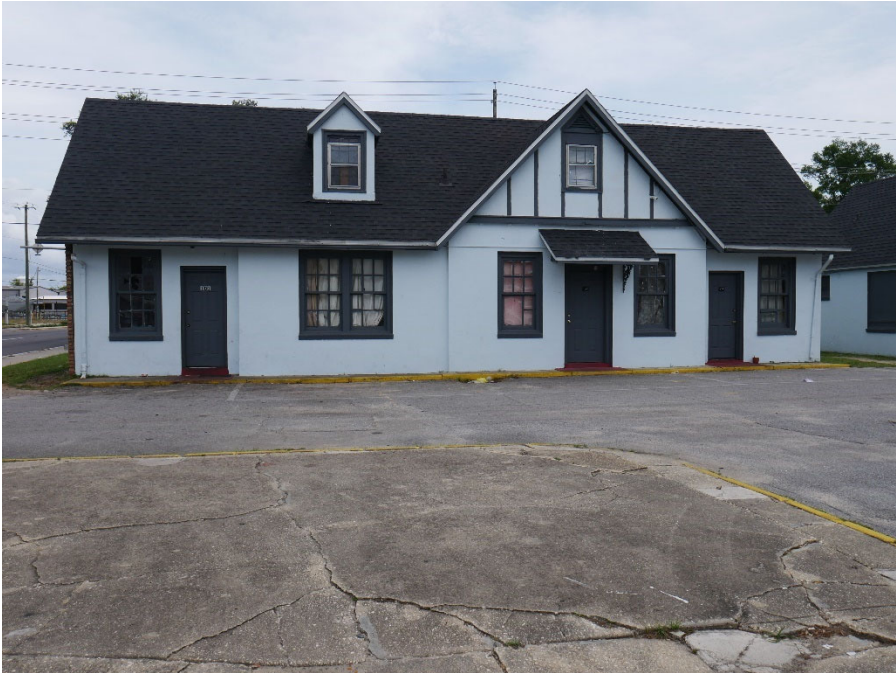
Front Exterior of Building with Units 101, 102, 103 and 104
