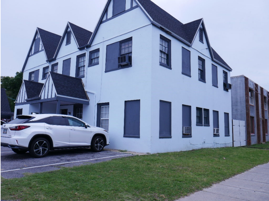
Front Exterior View of Office/Apartment and Upstairs Lodging Units
