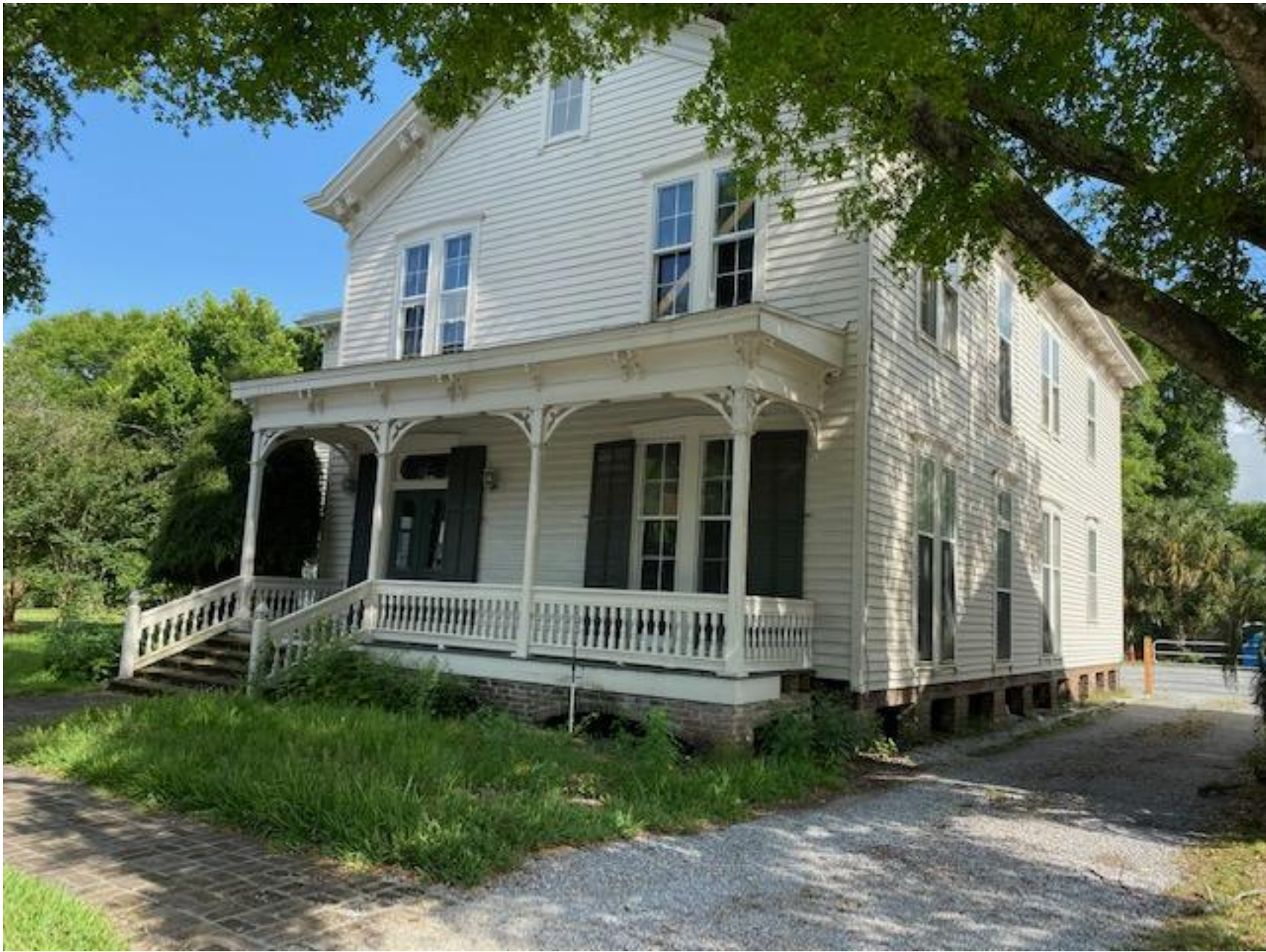
226 Government Existing Elevation Looking at East Side
