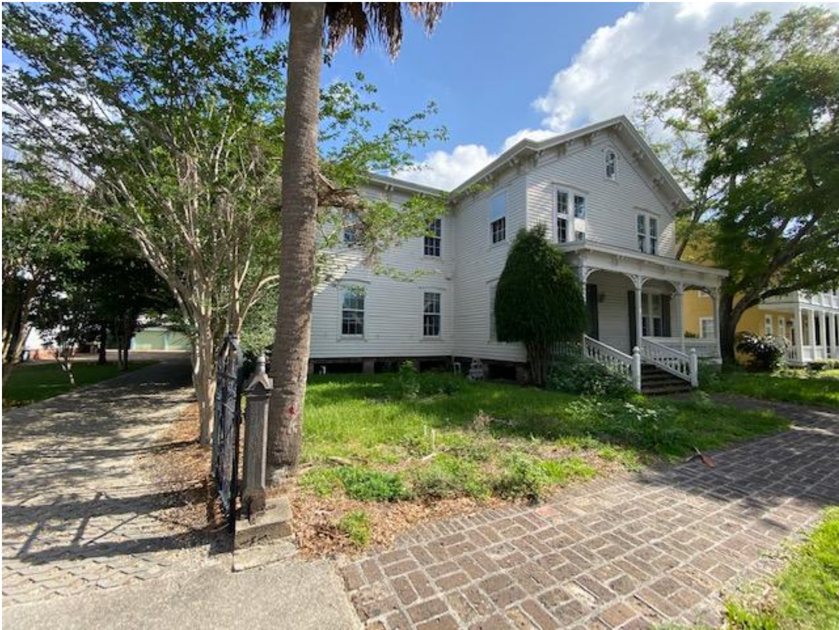
226 Government Existing Elevation Looking towards West Side
