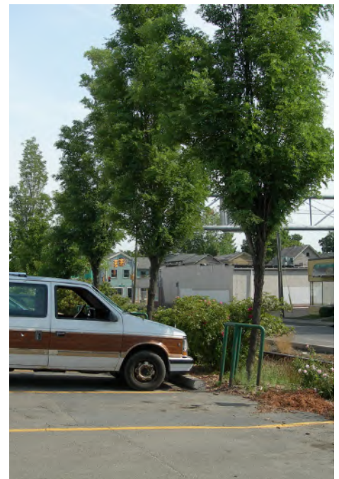
Fig. 1.15 In this parking lot, there is only a 2 foot opening for tree planting. Here CU-Structural Soil™ was installed parallel to railroad tracks, 12' wide and 36" deep. With such a narrow opening, there is no reason to use a planting mix other than CU-Structural Soil™ around the tree ball.
