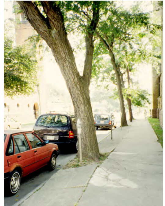
Fig. 1.10 Sidewalk heaving caused by superficial tree root growth, Ithaca, NY
