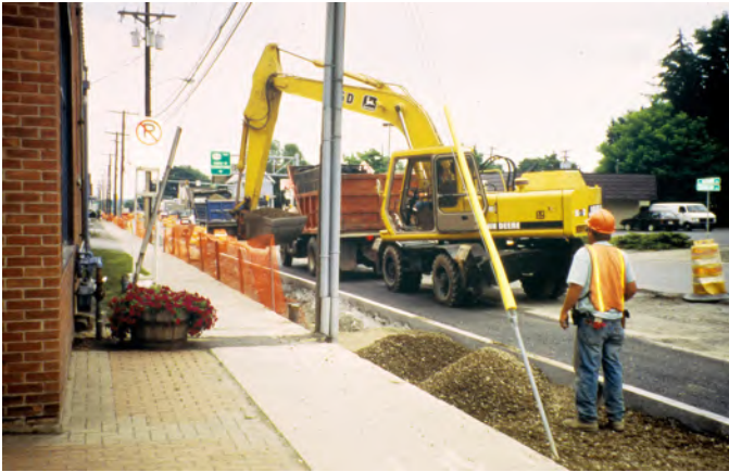
Fig.1.9 Installing CU-Structural Soil™ in Ithaca, NY in 1997
