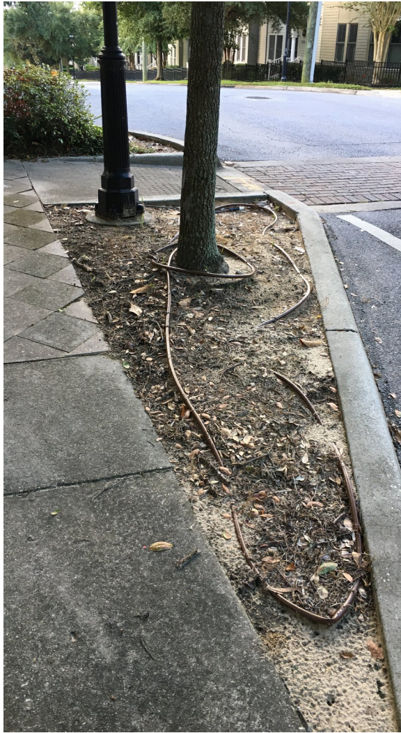
Conditions: Landscape in poor condition, irrigation lines exposed, power washing needed.
