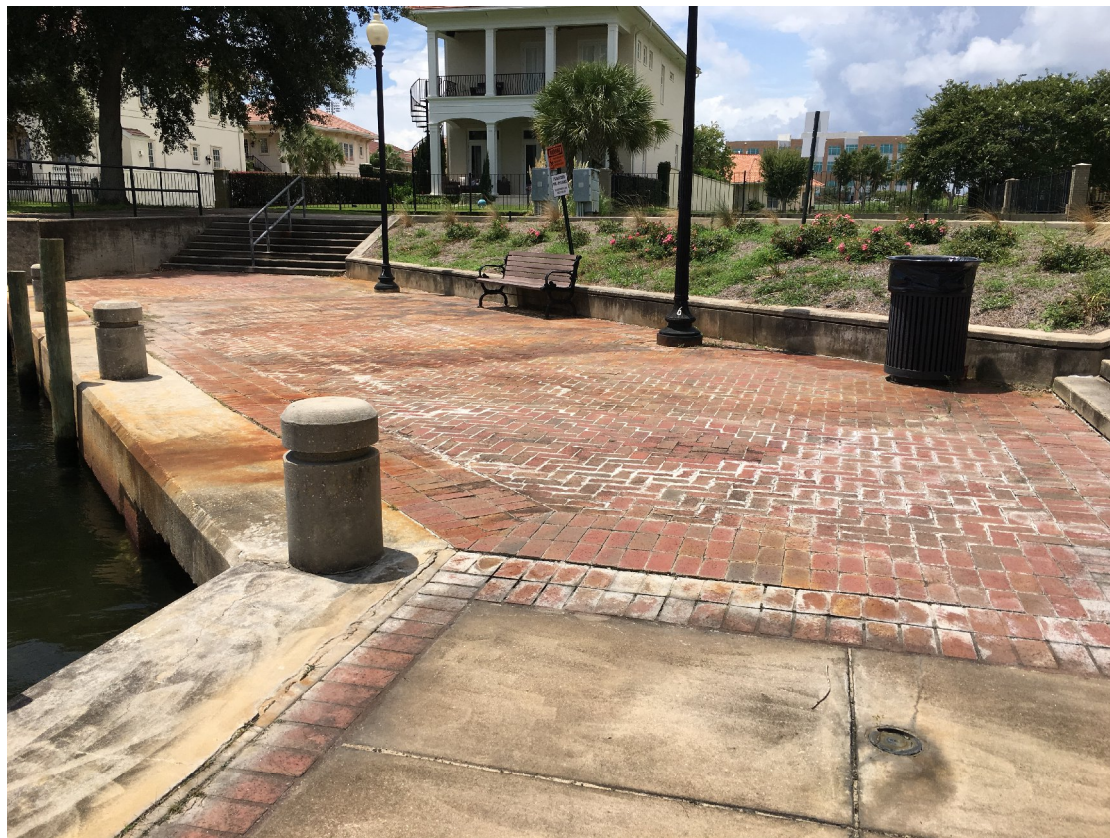
Conditions: Promenade sinking, corrosion, pavers lifting, landscape in poor condition
