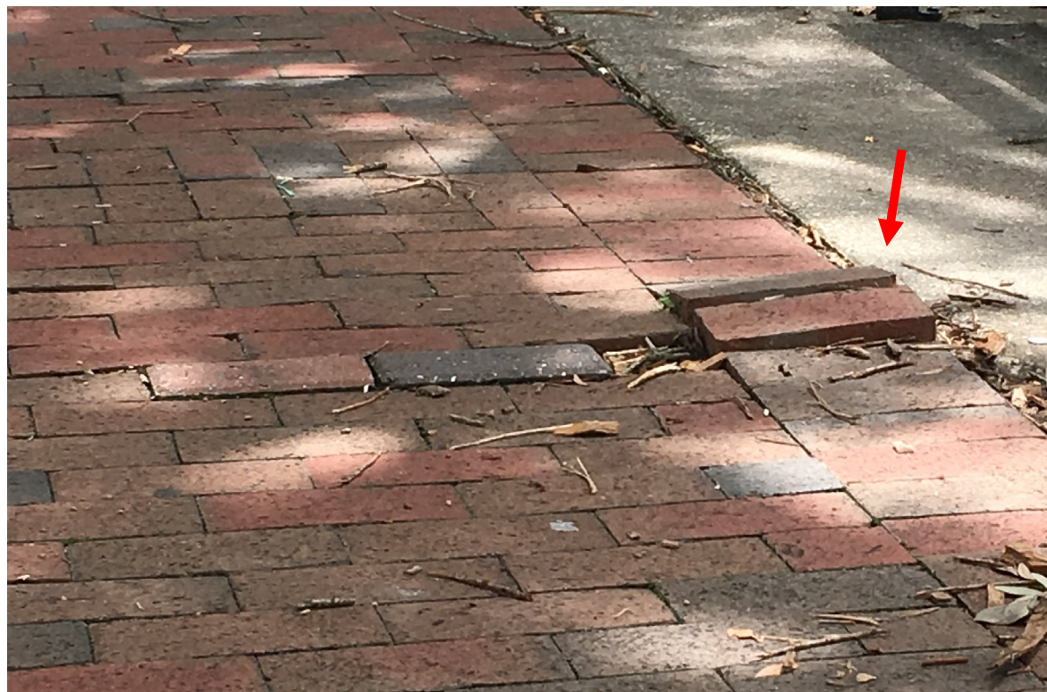
Conditions: Paver lifting, trees/landscape in poor condition
