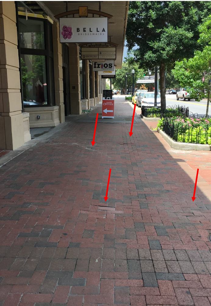
Conditions: Major pavement buckling and lifting along segment length.
