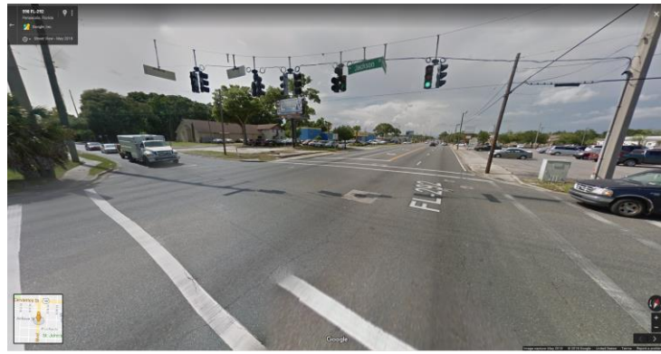
Jackson Street Intersection at Pace Boulevard Showing Need to Refresh Crosswalk Paint
