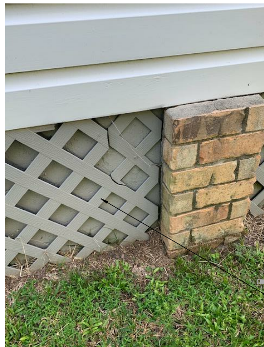
EXISTING WOOD BASE LATTICE WORK & FAUX BRICK PIER - TO BE DUPLICATED ON PROPOSED HOUSE ADDITION'S EXPOSED FOUNDATION
