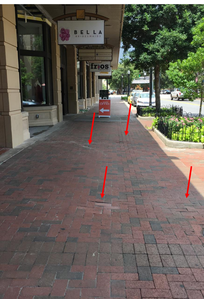
Conditions: Major pavement buckling and lifting along segment length.
