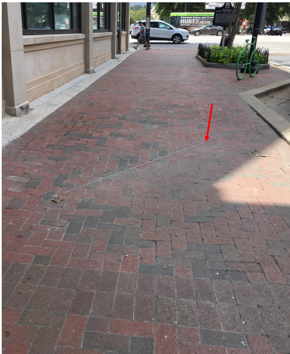
Conditions: Major pavement buckling and lifting along segment length.
