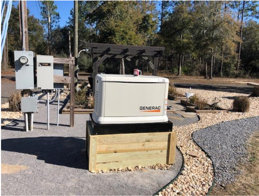
Black-Coated Aluminum Platform with Generac Generator
