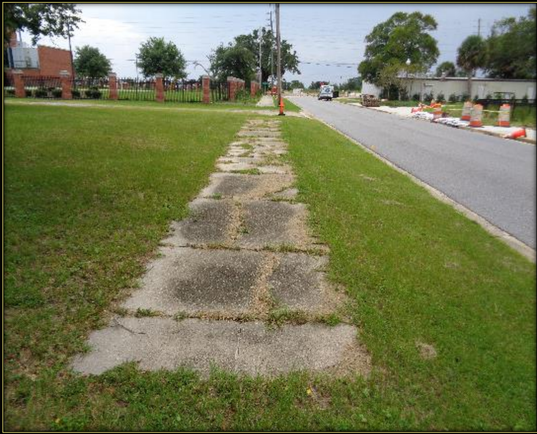
Sidewalk disconnected, broken, vegetation
