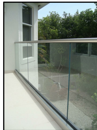
GLASS GUARDRAIL @ ROOF TERRACE & BALCONIES
