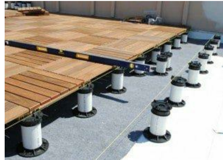
ROOF TERRACE: BY "TILE TECH" w/ SYTHETIC WOOD FIBER FLOORING
