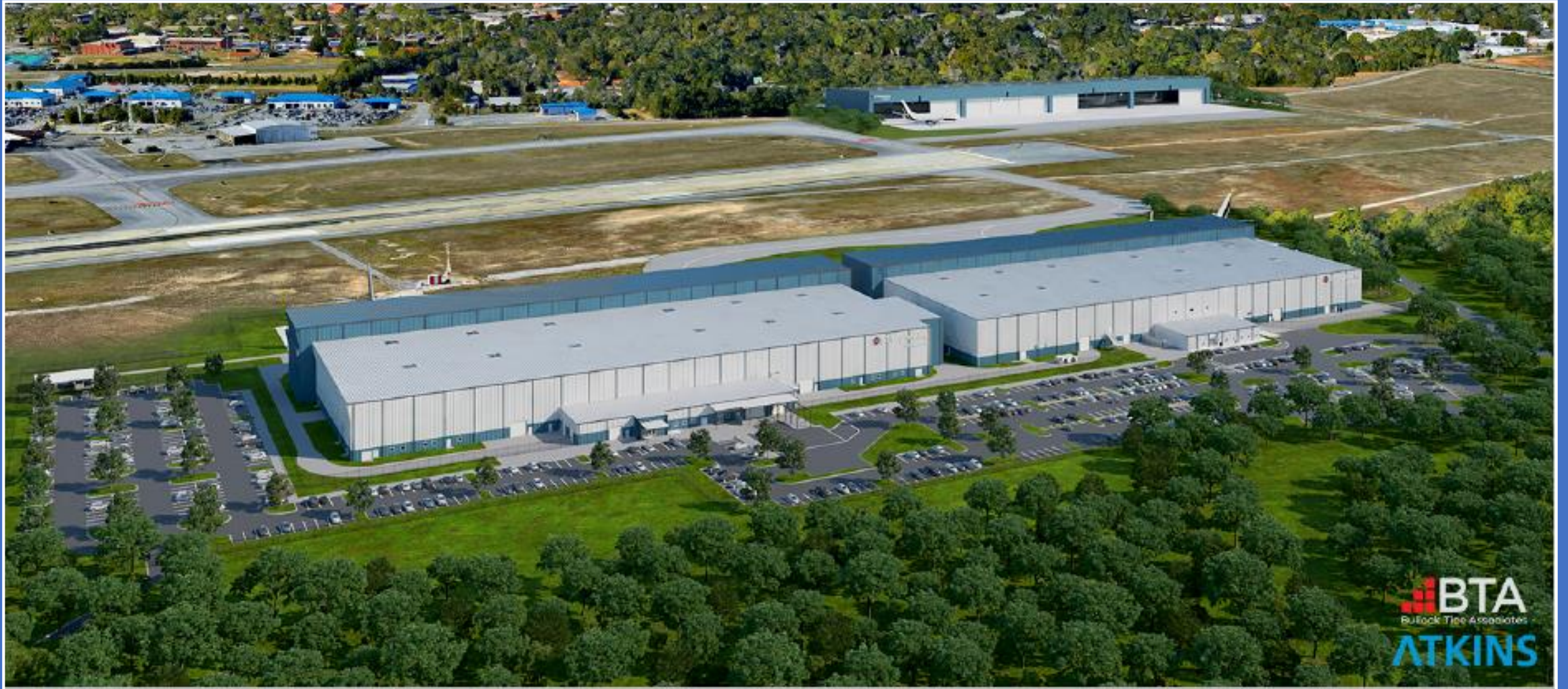
Hangar 2 concept – Landside, with approximately 21,000 sf Support Service Center (SSC) including warehousing, shops, vertical lift modules for automated parts and materials handling.
