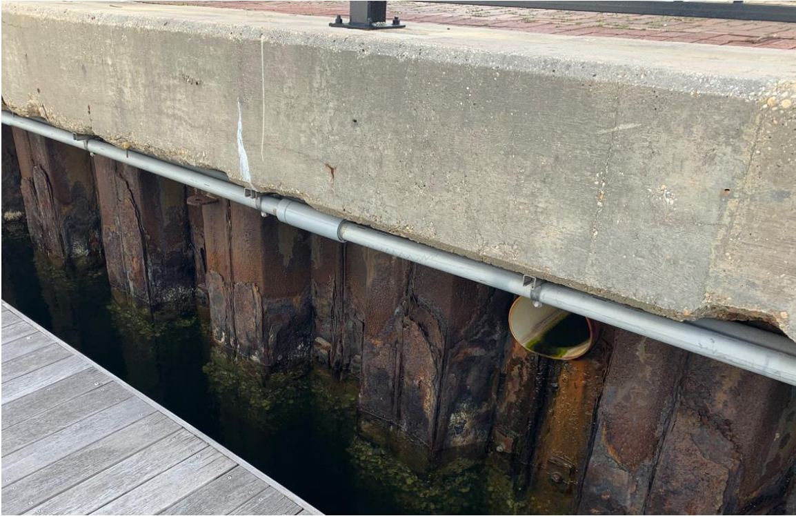
Photo 9 – Severe corrosion in east wall (Palafox Side)
