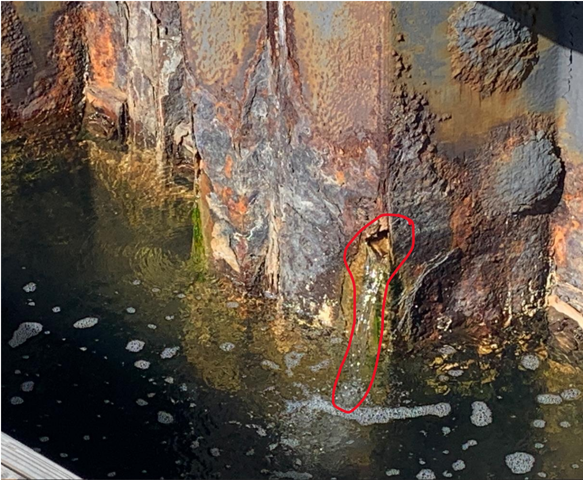
Photo 2 – Hole in west wall with water coming through (Port Royal Side)
