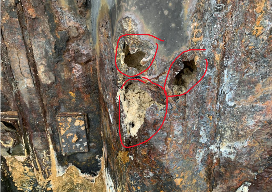
Photo 8 – Severe corrosion & Holes in west wall (Port Royal Side)
