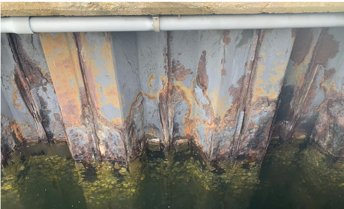
Photo 10 – Severe corrosion in east wall (Palafox Side)
