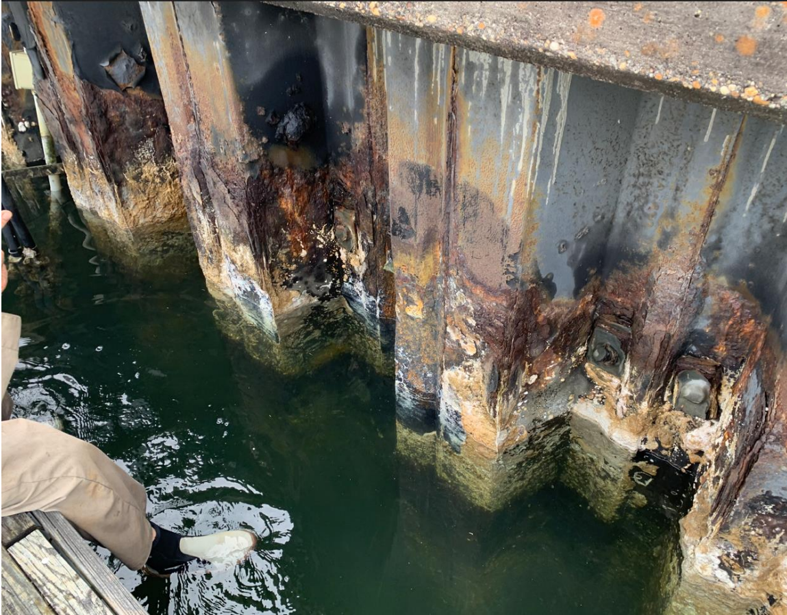
Photo 6 – Severe corrosion in west wall (Port Royal Side)
