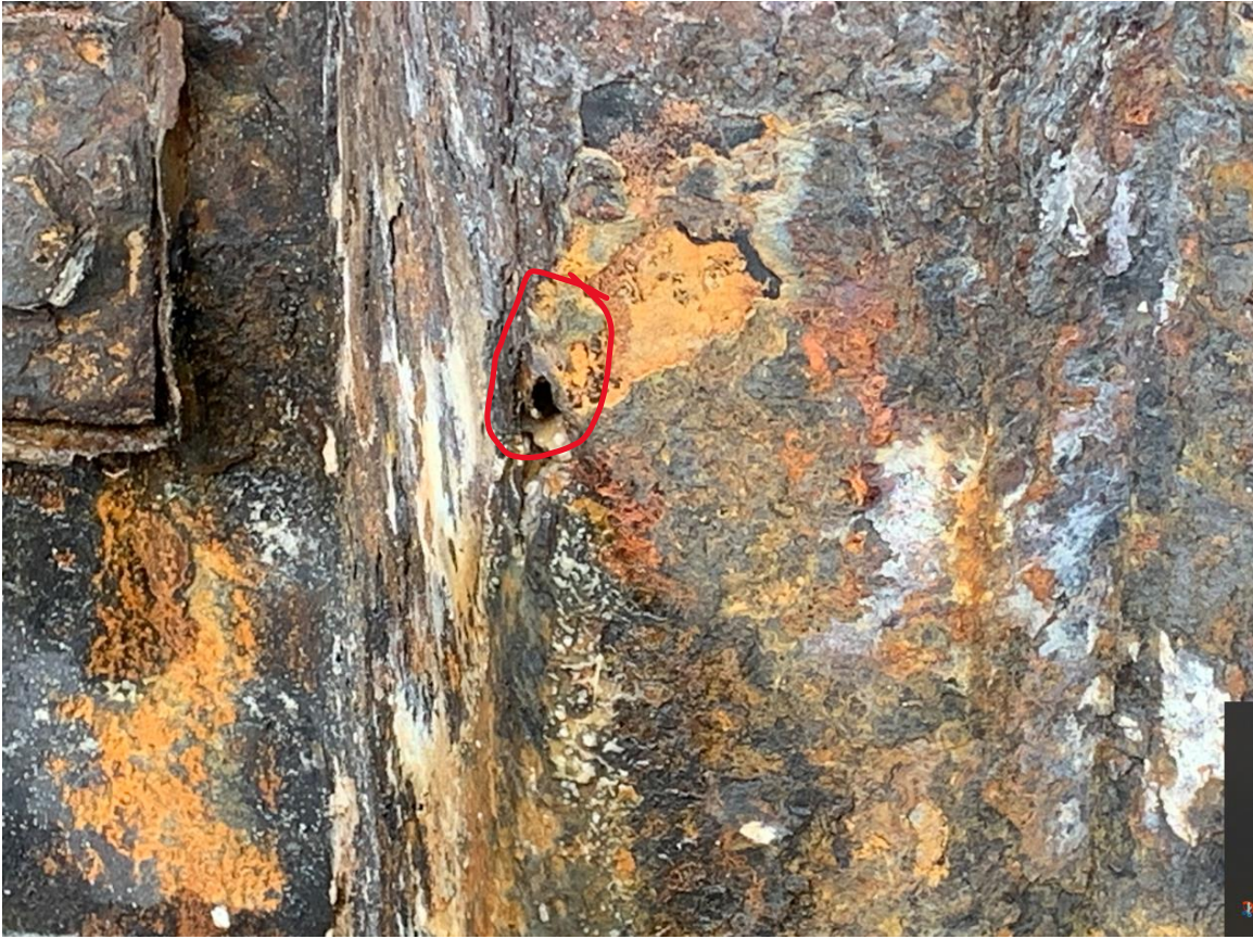
Photo 5 – Severe corrosion & small hole in west wall (Port Royal Side)
