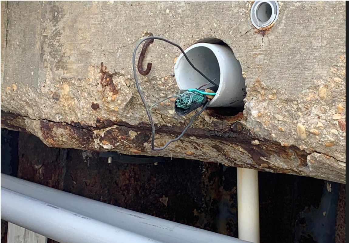
Photo 15 – Severe corrosion in east concrete cap rebar resulting in spalls along bottom (Palafox Side)
