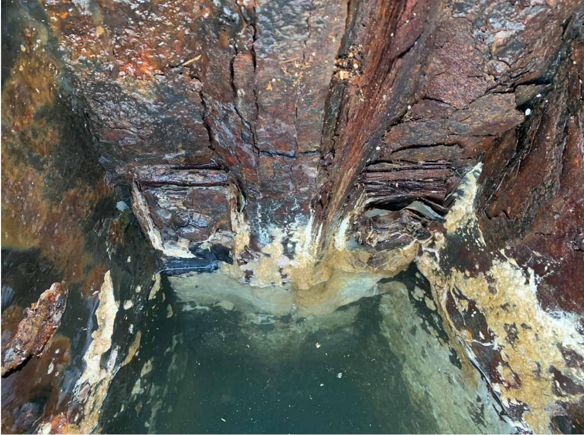
Photo 3 – Severe corrosion in west wall (Port Royal Side)
