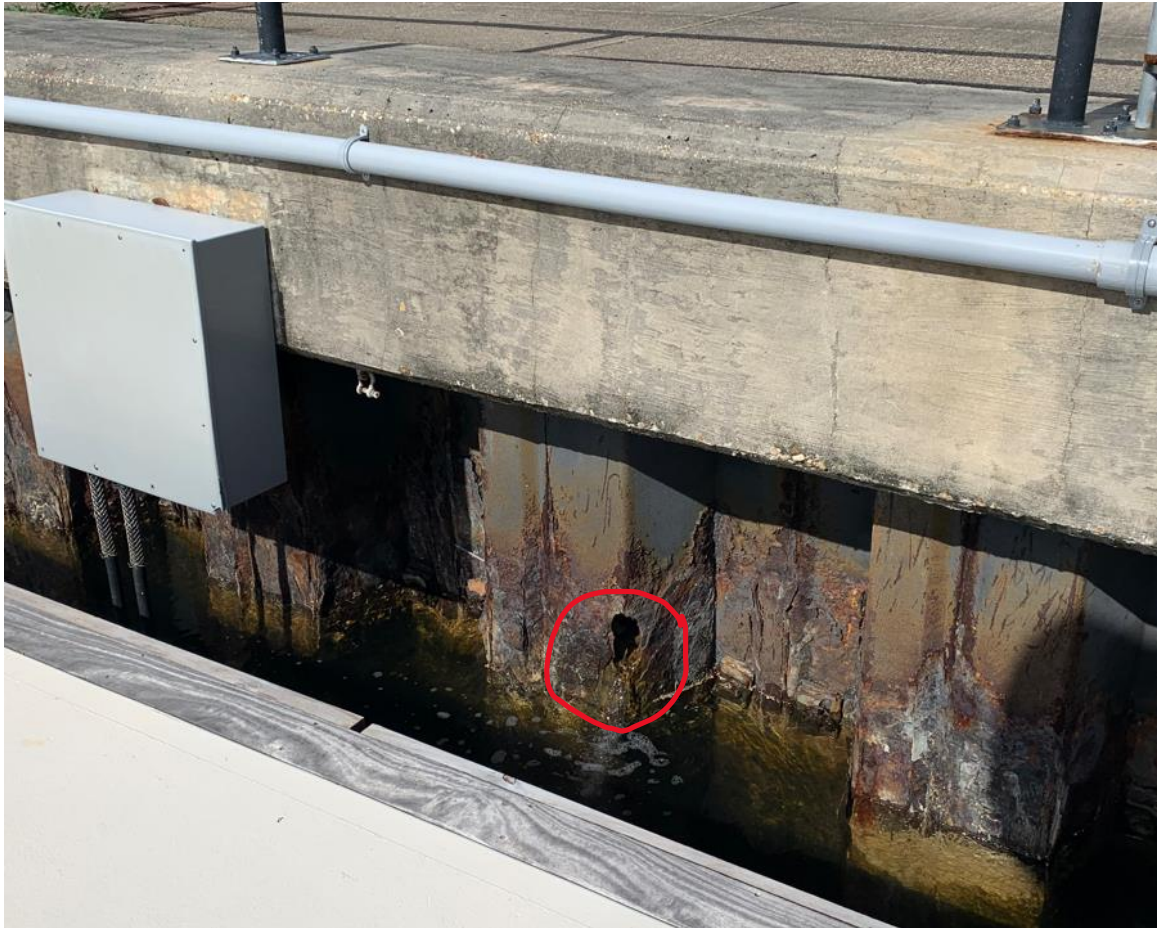
Photo 1 – Hole in west wall (Port Royal Side)
