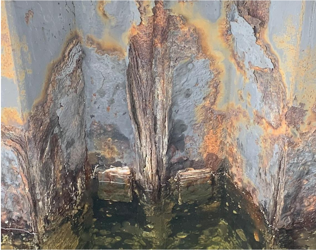
Photo 11 – Severe corrosion in east wall (Palafox Side)
