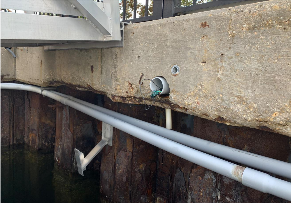
Photo 14 – Severe corrosion in east concrete cap rebar resulting in spalls along bottom (Palafox Side)
