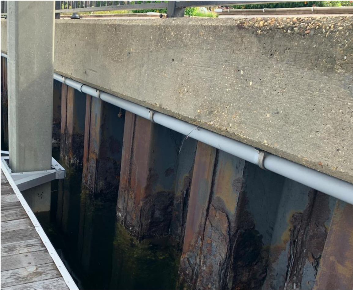
Photo 12 – Severe corrosion in east wall (Palafox Side)
