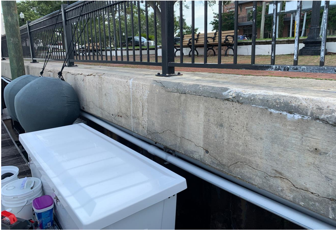
Photo 13 – Severe corrosion in east concrete cap rebar resulting in cracking (Palafox Side)
