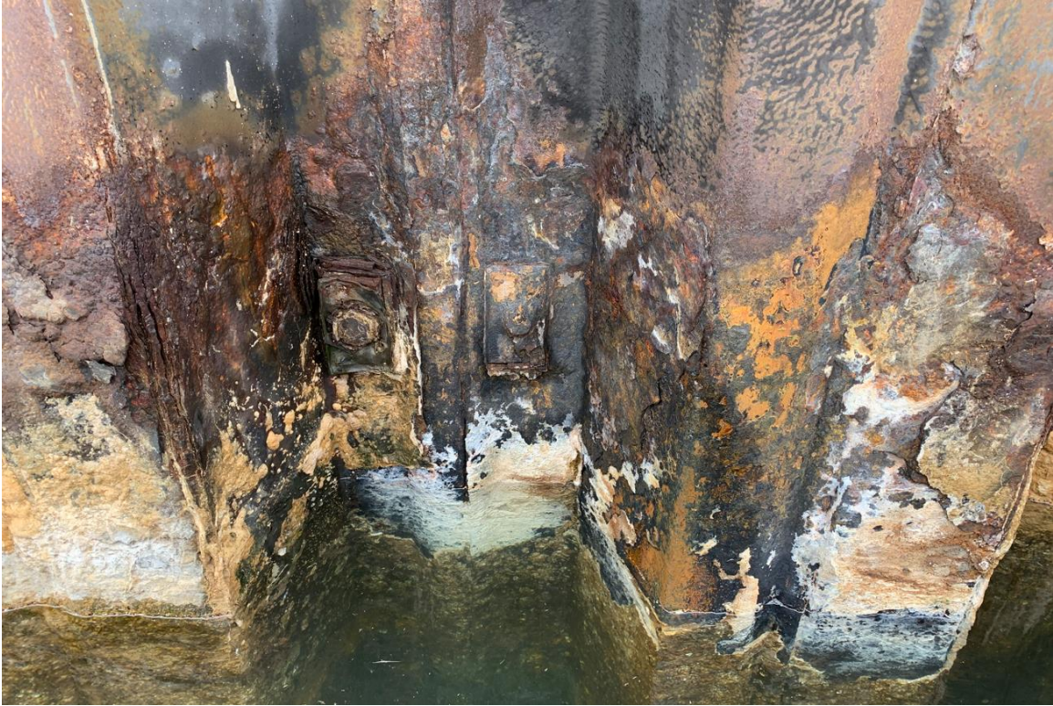
Photo 7 – Severe corrosion in west wall (Port Royal Side)
