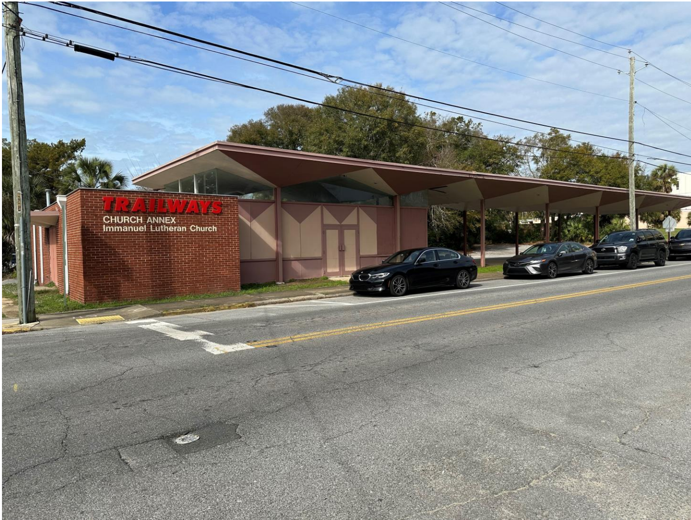
Immanuel Lutheran Church Overflor parking Northwest view
