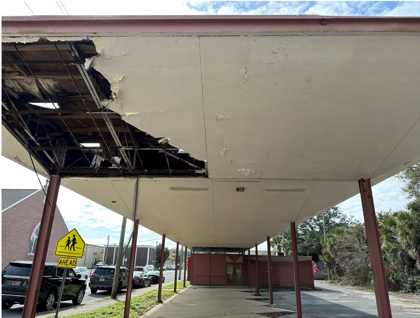
Immanuel Lutheran Church Overflor parking South view
