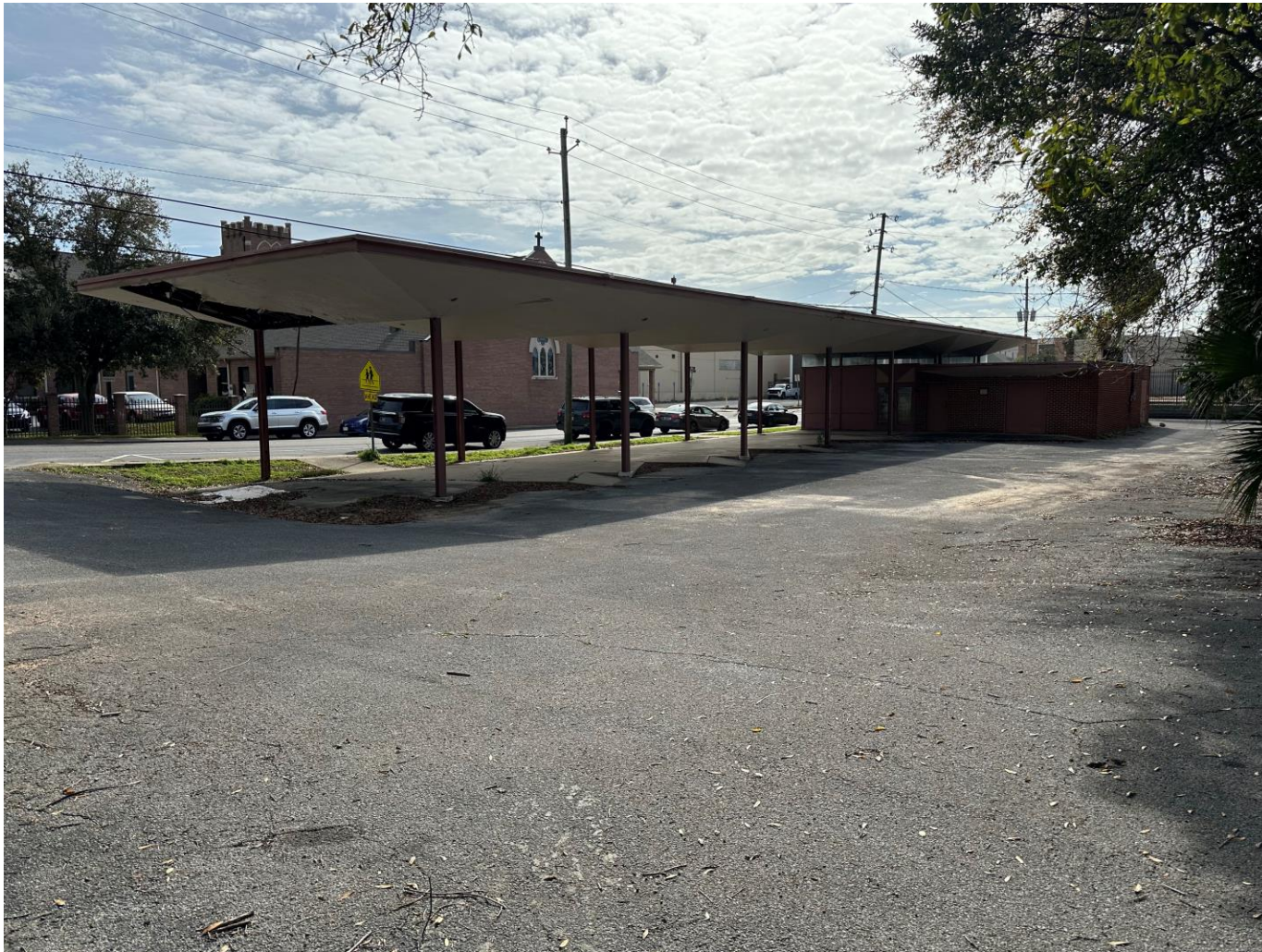
Immanuel Lutheran Church Overflor parking Southwest view
