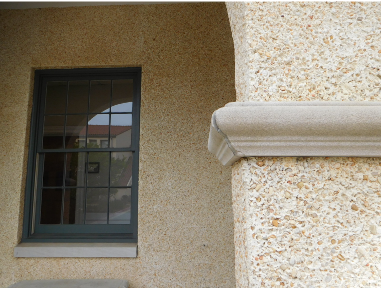
PHOTO DIPICTING EXISTING FINISHES TO MATCH TO FOR STUCCO, STRING COURSES AND KITCHEN WINDOW (SEE A7 FOR KITCHN WINDOW COLOR SELECTION)
