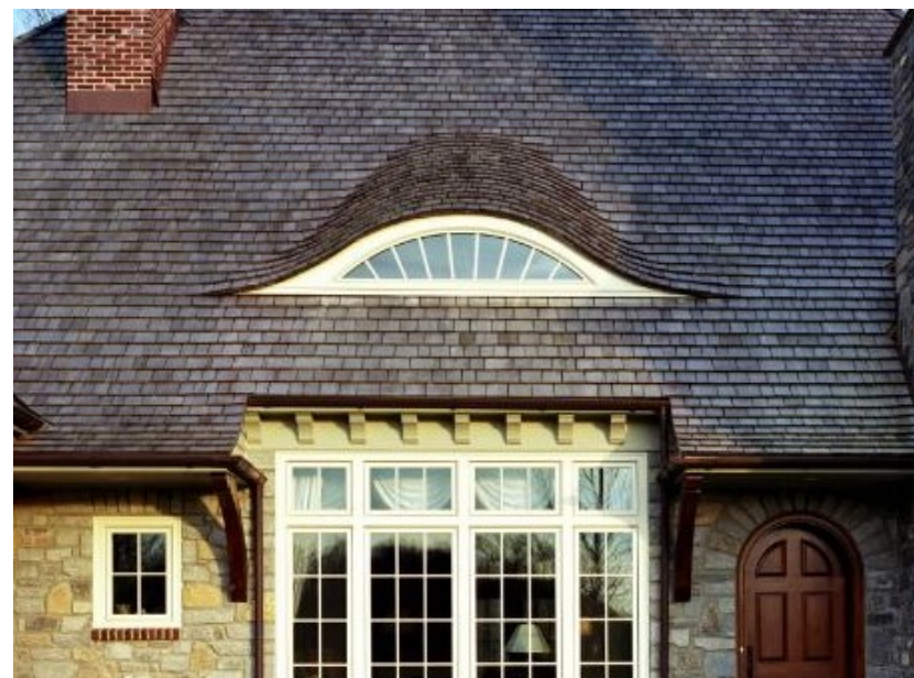
Example of eyebrow dormer window installed
