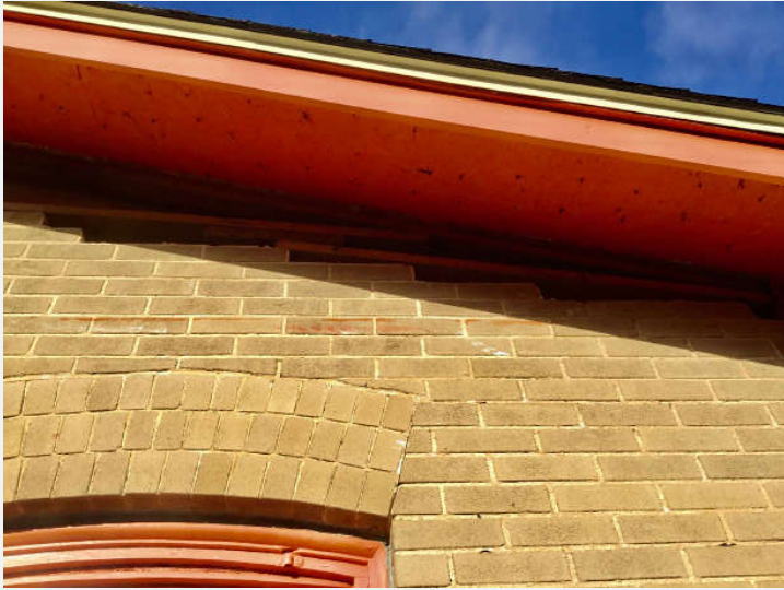
BRICK DAMAGE AT EAVES
