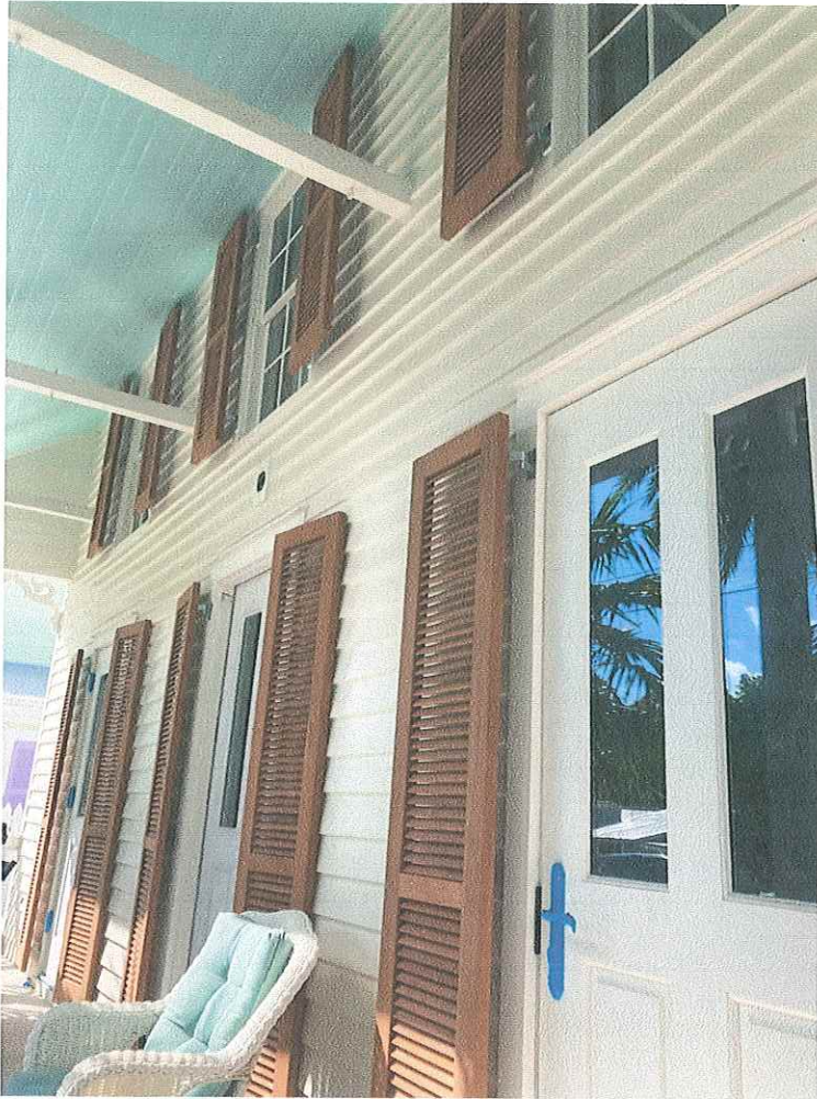
TYPICAL HINGED INSTALLATION STYLE FOR 314
