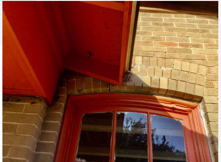
EXISTING ENTRY PORCH OBSCURES ORIGINAL BRICK DETAIL ABOVE WINDOW
