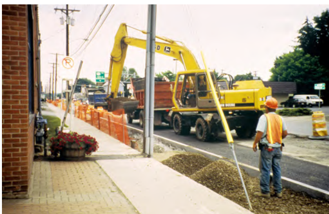
Fig.1.9 Installing CU-Structural Soil™ in Ithaca, NY in 1997
