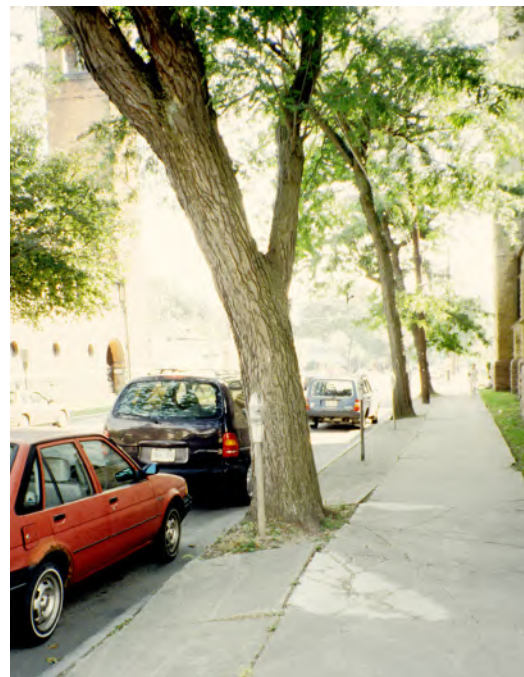
Fig. 1.10 Sidewalk heaving caused by superficial tree root growth, Ithaca, NY
