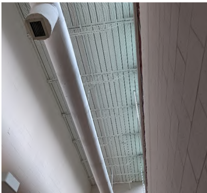
Figure 16: Roof Framing - Bar Joists - Vickrey Center Offices
