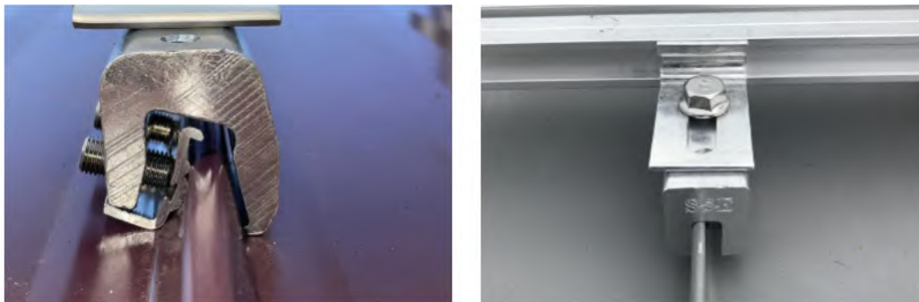
Figure 23: Standing Seam Metal Roof Clamp Mounts
