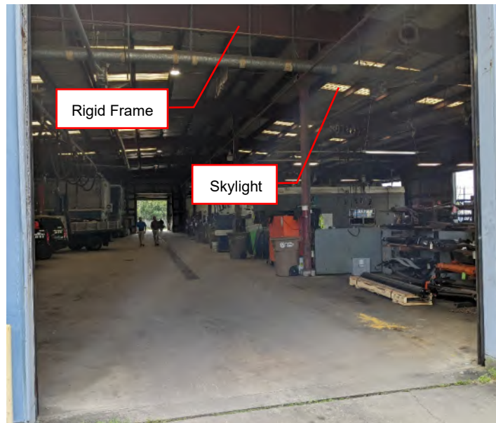
Figure 11: Roof Framing - Fleet Garage
