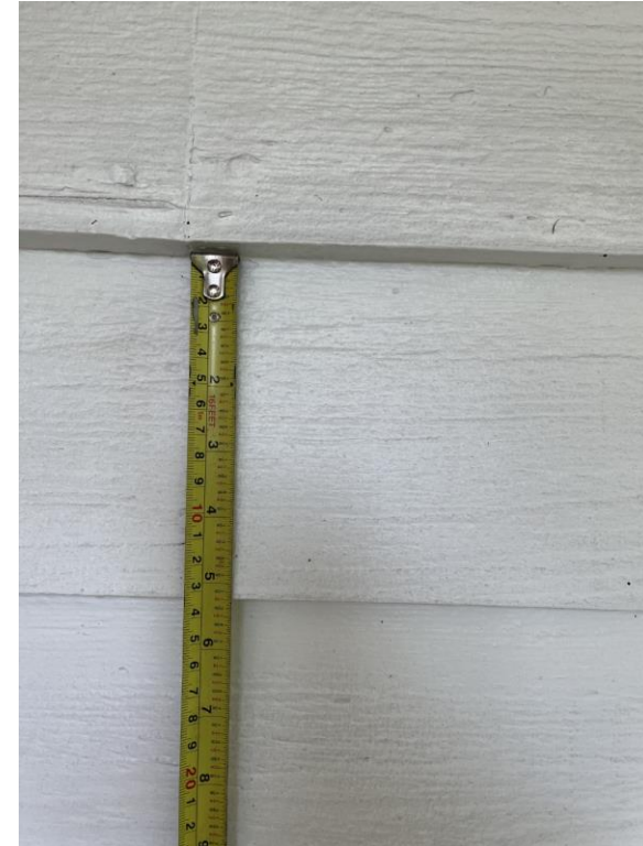
HARDI LAP SIDING 5.5" EXPOSER SMOOTH PAINTED WHITE TO MATCH HOUSE
