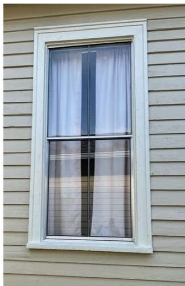
Replace (3) existing single hung wood windows to match existing design and color.
