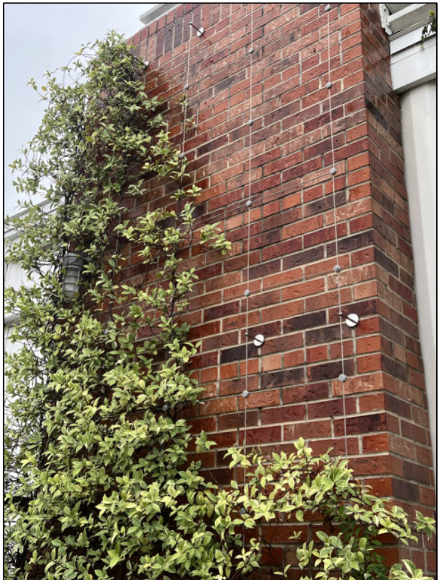
Option #2 Live Jasmine on Stainless Steel cable grid substrate
