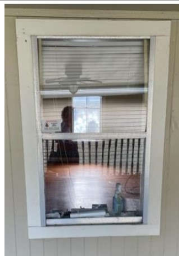
Replace (1) single hung wood window to match existing design and color.
