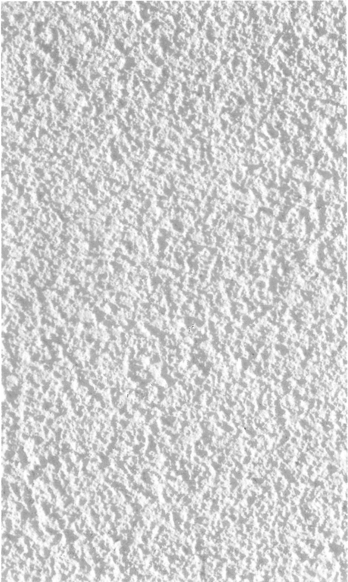
Foundation: Exposed block, sand finish stucco, natural (light gray) color.
