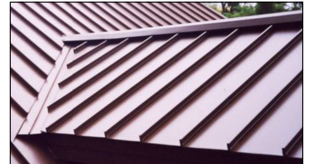
STANDING SEAM METAL ROOF ( profile example) BERRIDGE MFG. / COLOR: "DARK BRONZE" 12.75" T-LOCK / FLAT PANEL METAL ROOF (see spec on sheet A4)
